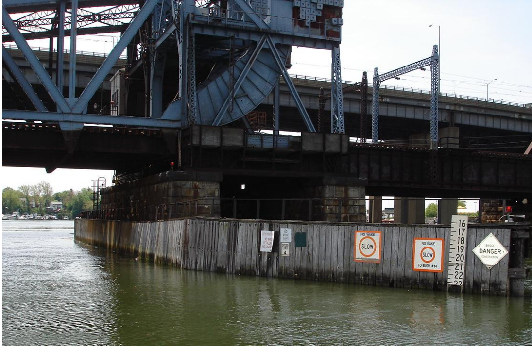
Figure 6.4.1a – Timber Fender System with navigation lights.
