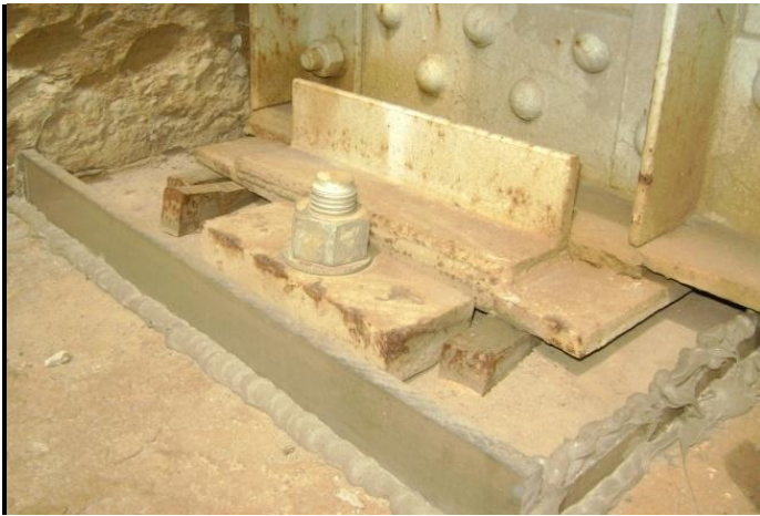
Figure 6.2.1s - Bearing shimmed and prepped for grouting
