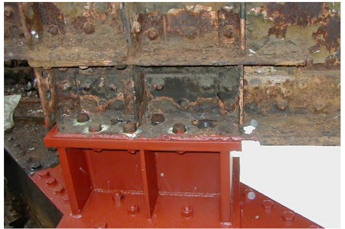
Figure 6.2.1n - Fixed bearing on top of a pier cap
