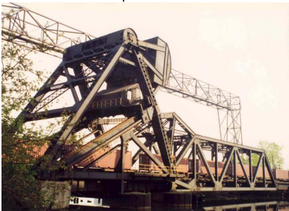
Figure 6.2.6.2c Strauss trunnion bascule - lowered position
