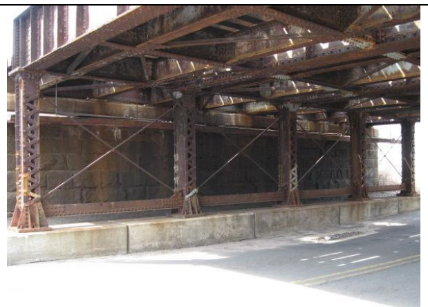
Figure 6.3.3d: Typical steel columns
