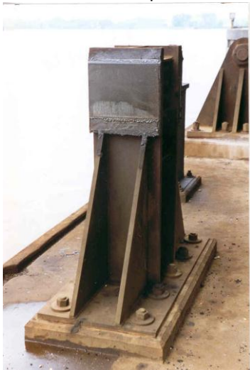
Figure 6.2.6.3k Lift span - centering device
