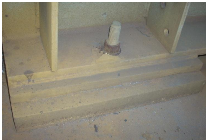
Figure 6.2.1i - Fixed plate bearing
