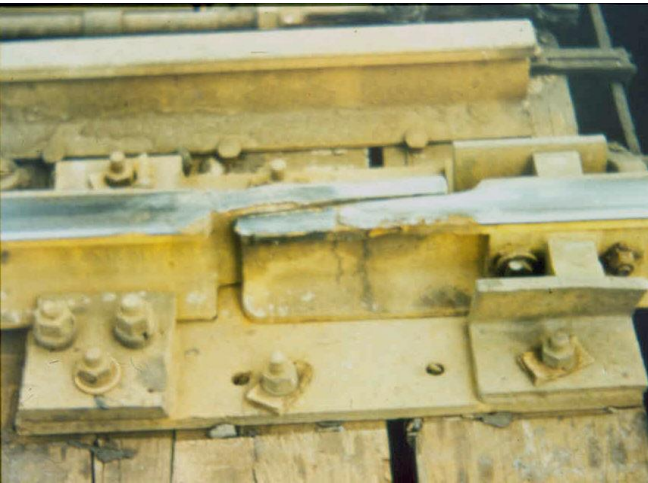
Figure 6.2.6.3w Two-piece miter rail worn points
