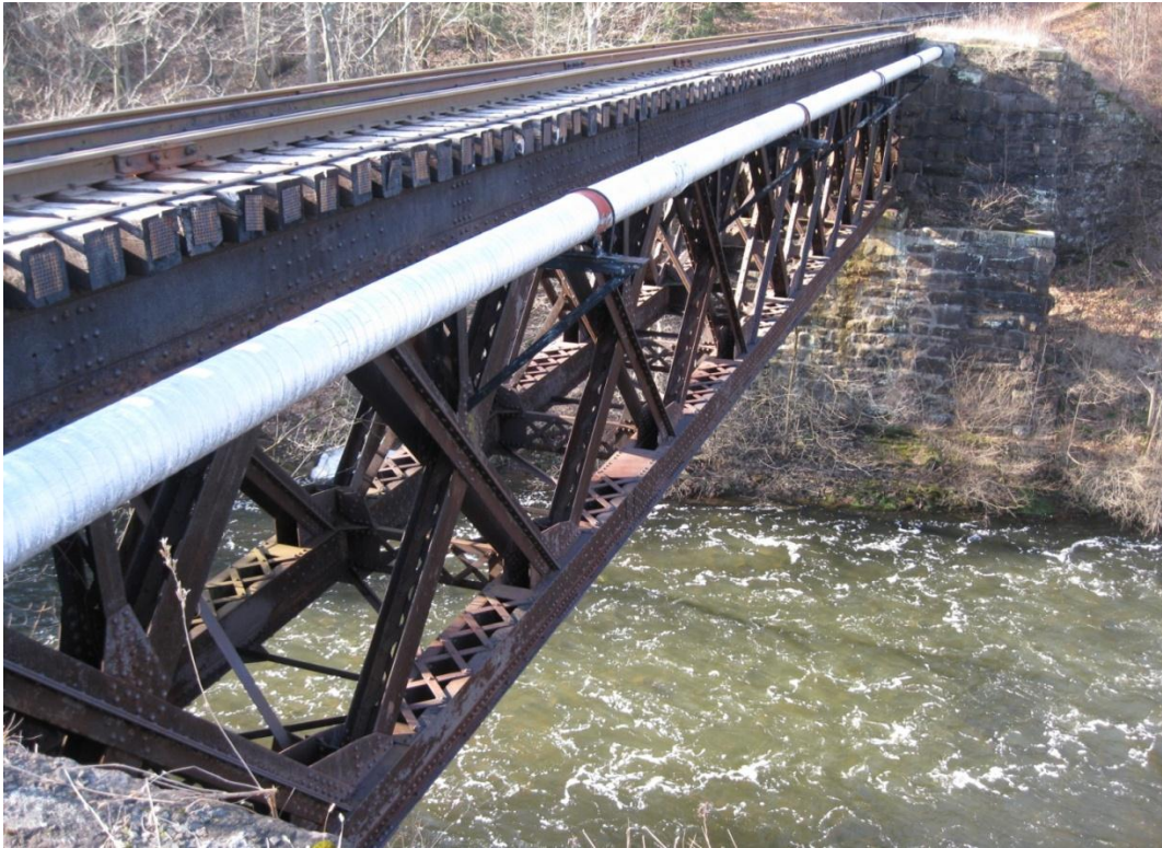
Figure 6.1.9a: Typical Bridge Utility Installation
