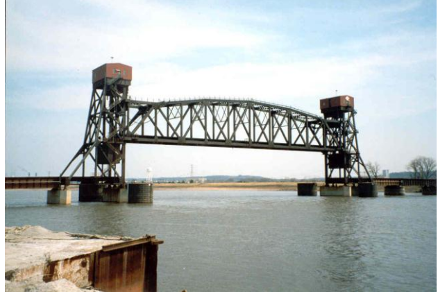
Figure 6.2.6.3b Vertical lift – raised position tower drive
