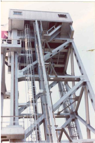
Figure 6.2.6.3v Tower access caged ladder and elevator
