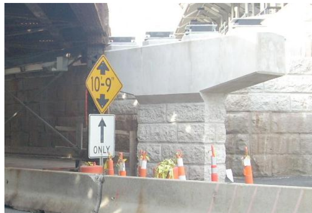
Figure 6.3.1d: Concrete Hammer head pier
