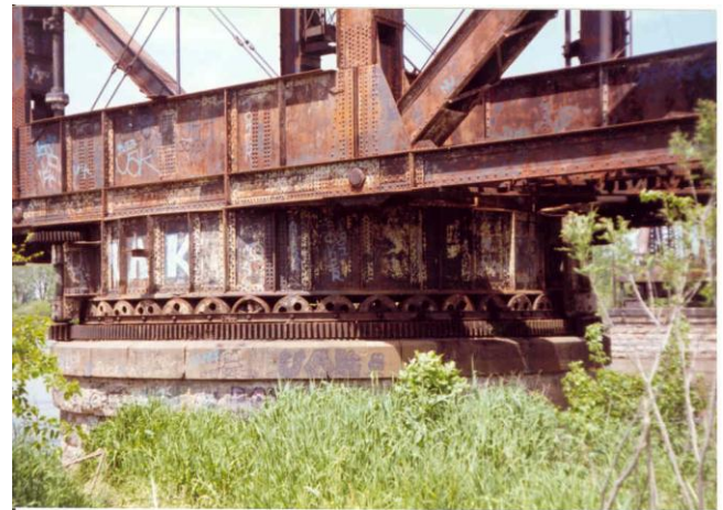
Figure 6.2.6.1f Swing span – rim support(load thru all wheels)
