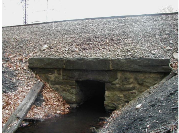
Figure 6.4d: Rail top box culvert
