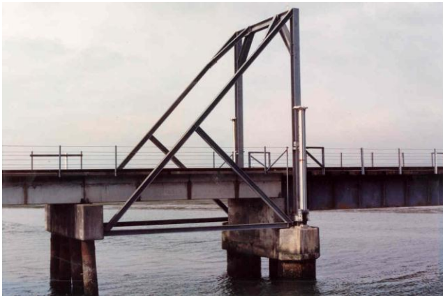
Figure 6.2.6.3e Vertical lift – hydraulic lift - infrequent openings
