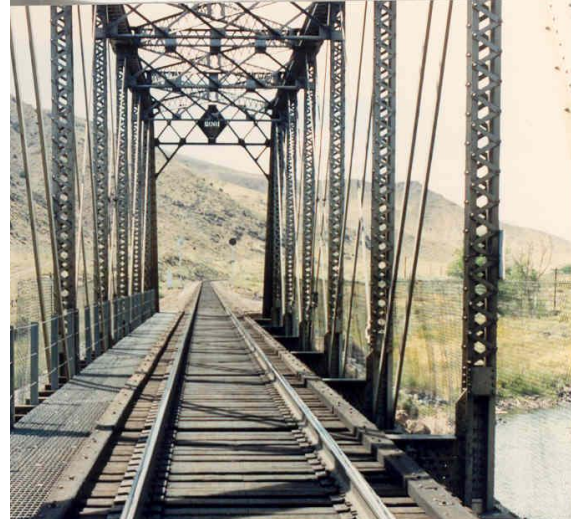
Figure 6.2.5b Pratt Truss – end view
