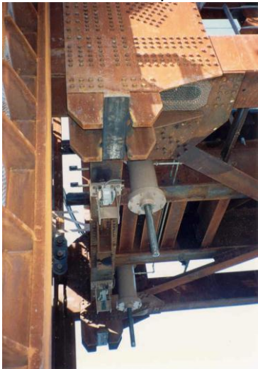
Figure 6.2.6.3l Sheave - trunnion bearing assembly
