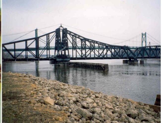
Figure 6.2.6.9b Fender system lining the channel
