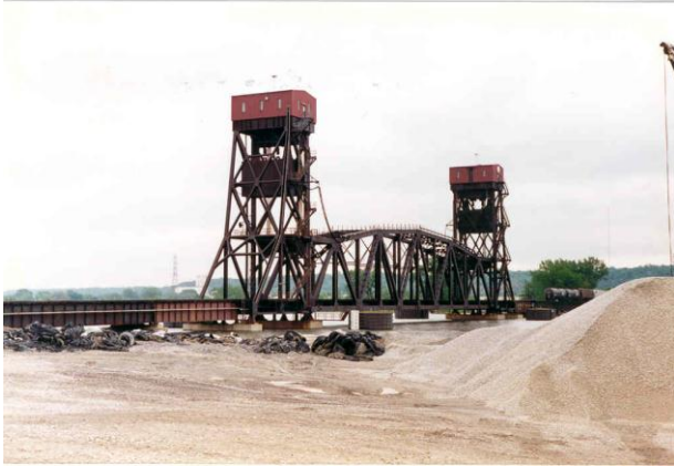
Figure 6.2.6.3a Vertical lift – lowered position tower drive
