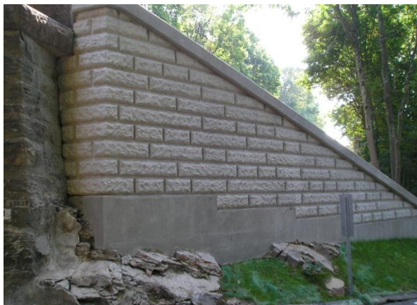
Figure 6.3.1c: Concrete Wingwall with decorative form liner
