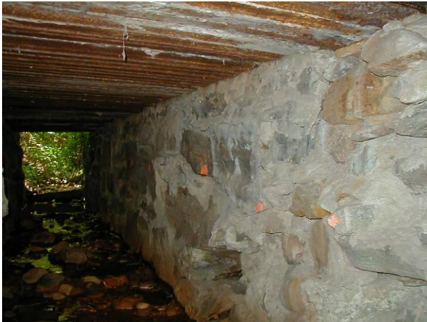
Figure 6.4e: inside a typical rail top box culvert
