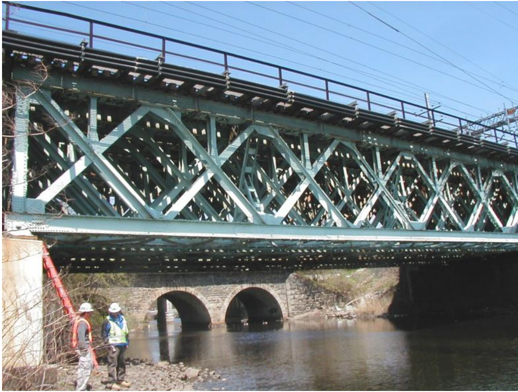
Figure 6.2.4c – Deck Truss Bridge.
