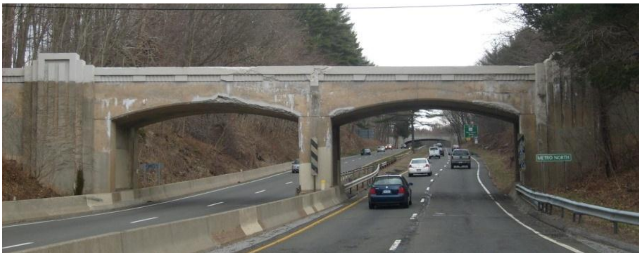
Figure 6.2.2.4-a: A Closed Spandrel Reinforced Concrete Arch Bridge
