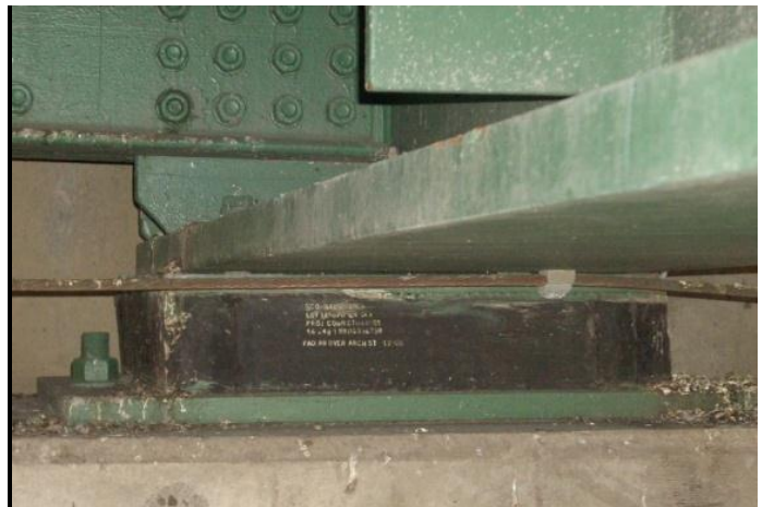
Figure 6.2.1l - Expansion elastomeric bearing
