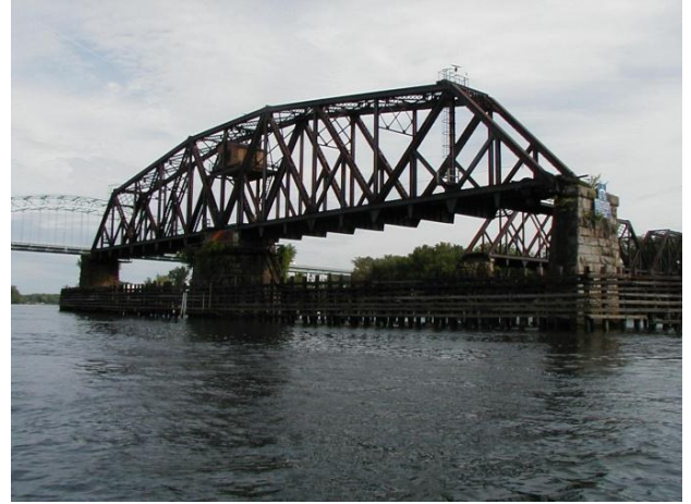
Figure 6.2.6.1b Swing span – truss Operator/Control House with good vision of channel
