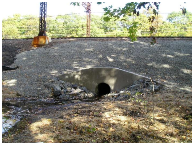
Figure 6.4b: Concrete pipe culvert
