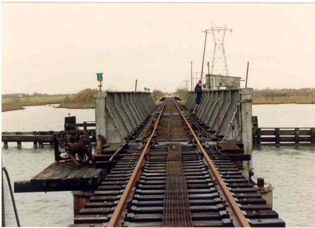
Figure 6.2.6.1c Swing span- girder closed position
