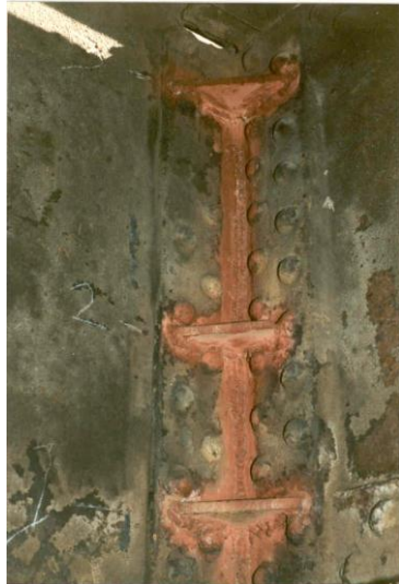
Figure 6.2.5k Reinforced stringer – floorbeam connection due to movement in truss members
