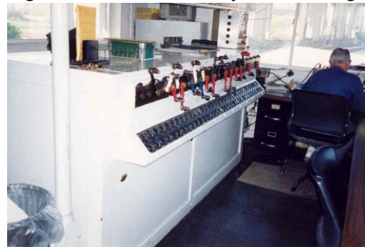
Figure 6.2.6.4d Operator's House interior
