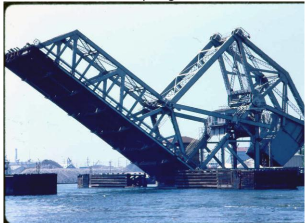
Figure 6.2.6.2d Strauss trunnion bascule - partially raised (note member parallelogram)
