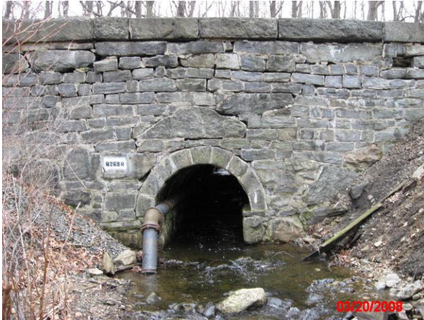
Figure 6.4c: Masonry arch culvert
