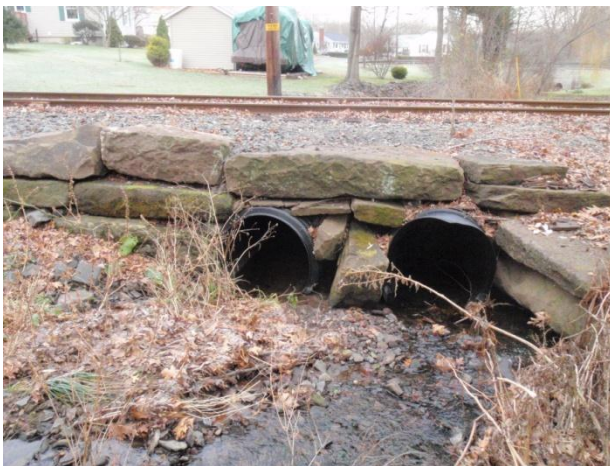
Figure 6.4a: Twin corrugated plastic pipe culvert
