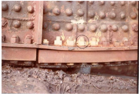
Figure 6.2.6.2g Rolling bascule - segment girder track
