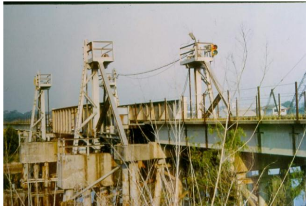
Figure 6.2.6.3f Vertical lift – screw jack lift
