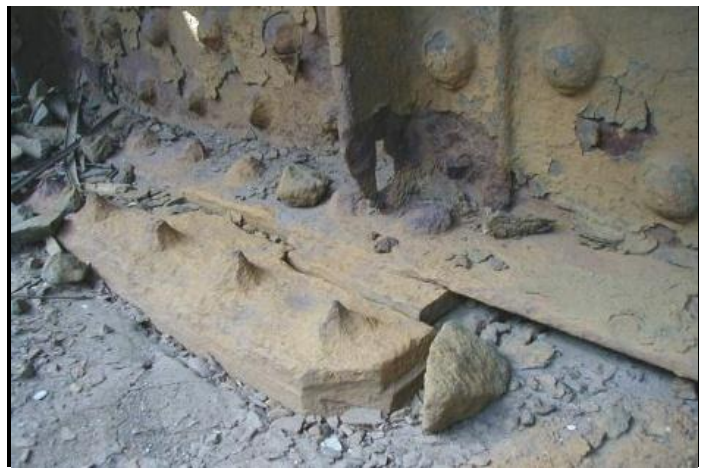
Figure 6.2.1j - Expansion sliding plate bearing
