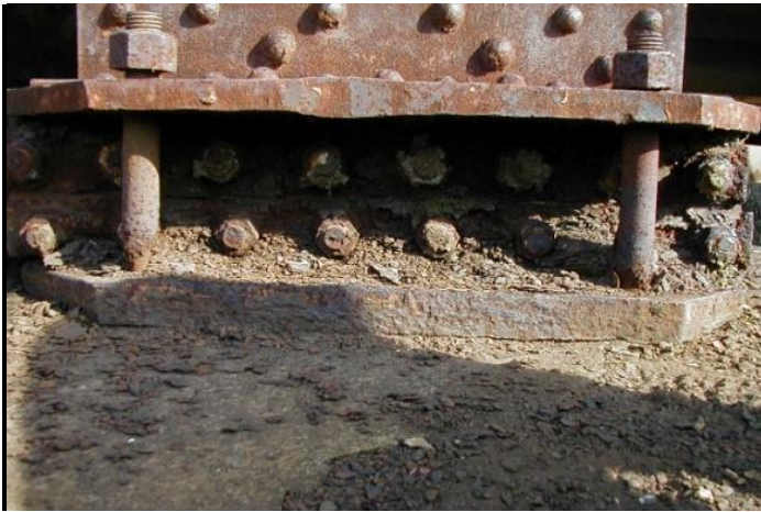
Figure 6.2.1m - Expansion roller bearing
