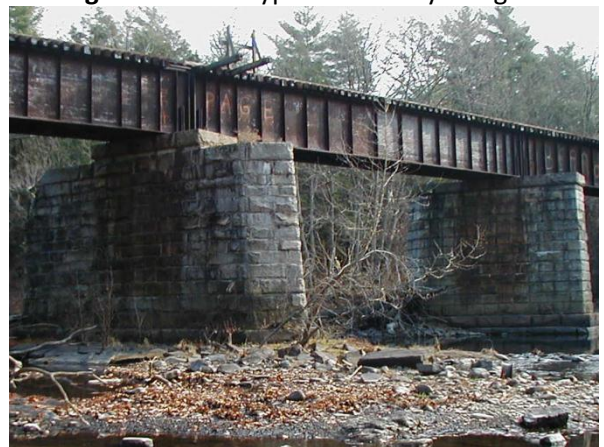
Figure 6.3.2d: Typical Masonry Piers
