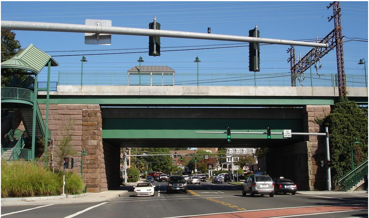
Figure 6.2.3.2.2b: Typical Multi-Girder Superstructure
