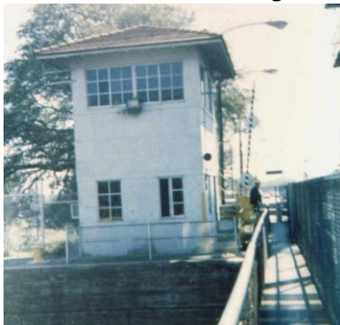
Figure 6.2.6.4c Operator's House 1 st floor – electrical - no alternative escape
