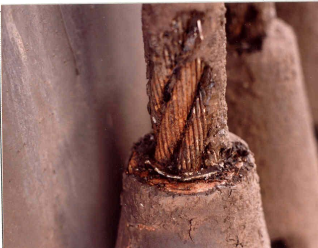
Figure 6.2.6.3q Counterweight ropes - raised spelter at socket - normal conditions
