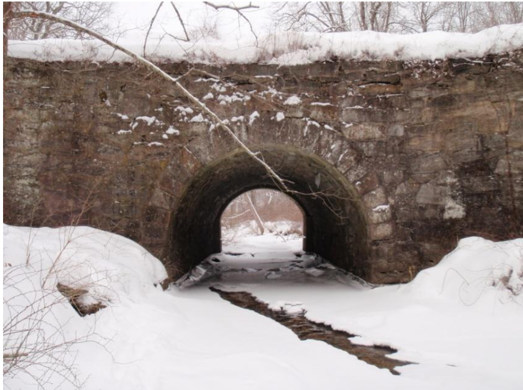
Figure 6.2.8b – Stone Masonry Arch
