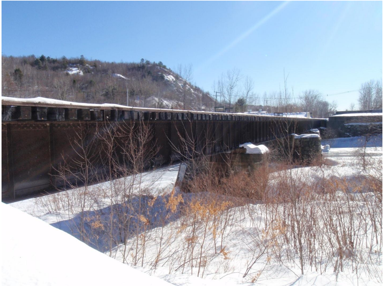
Figure 6.2.3.2.1-a: Typical Deck Plate Girder Superstructure
