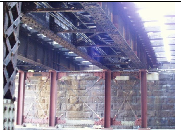
Figure 6.3.3b: Steel Column Supported Deck Plate Girders
