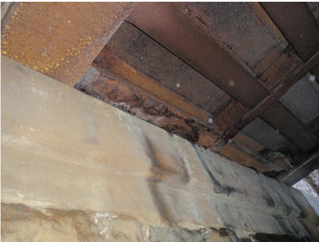
Figure 6.1.3.3a: Underside of Ballasted Metal Deck
