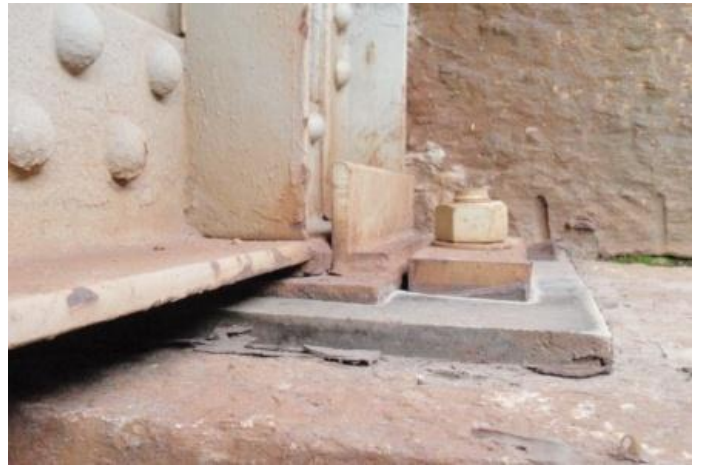
Figure 6.2.1t - Shimmed and grouted bearing
