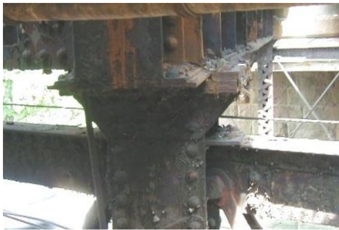
Figure 6.2.1o - Fixed bearing on top of a pier column
