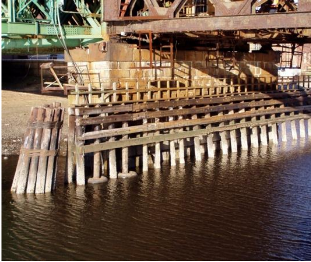
Figure 6.2.6.9g Typical fender system
