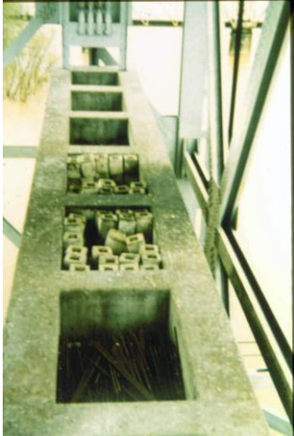
Figure 6.2.6.3t Counterweight balance pockets – weights not uniformly distributed
