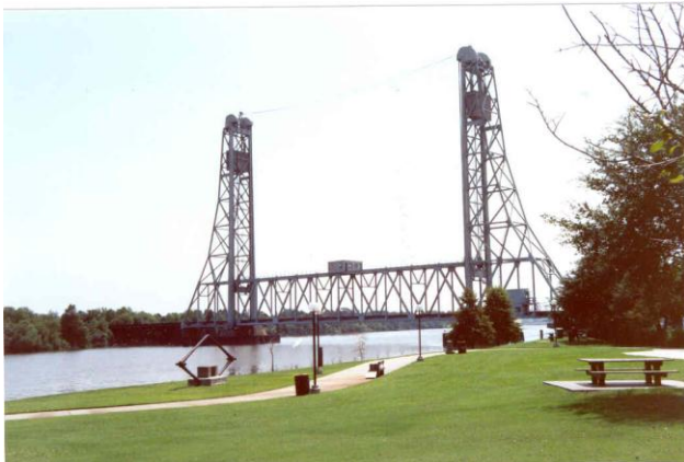
Figure 6.2.6.3c Vertical lift – lowered position span drive
