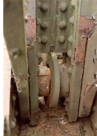
Figure 6.2.5h Pin and counter wear
