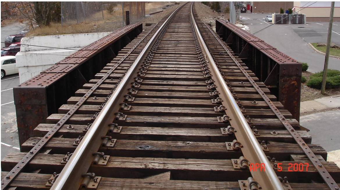
Figure 6.1.2b: Open deck on a Through Girder Bridge
