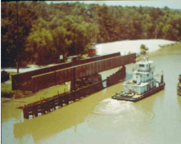
Figure 6.2.6.9a Fender system lining the channel
