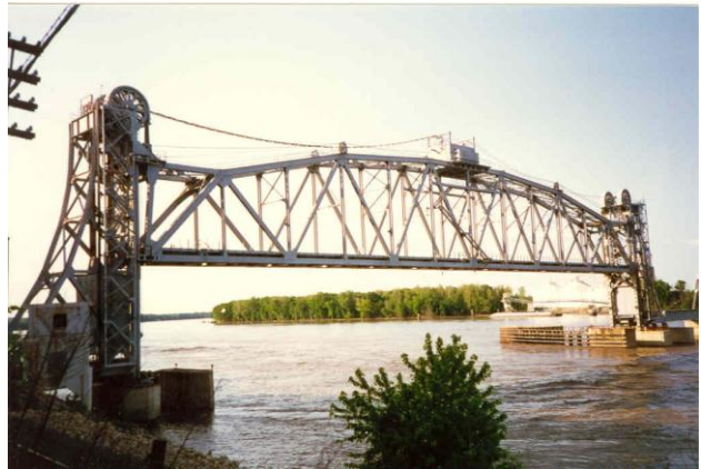
Figure 6.2.6.3d Vertical lift – raised position span drive
