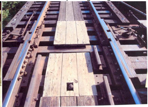
Figure 6.2.6.2p Strauss type bascule - operating strut with rack operating strut guide
