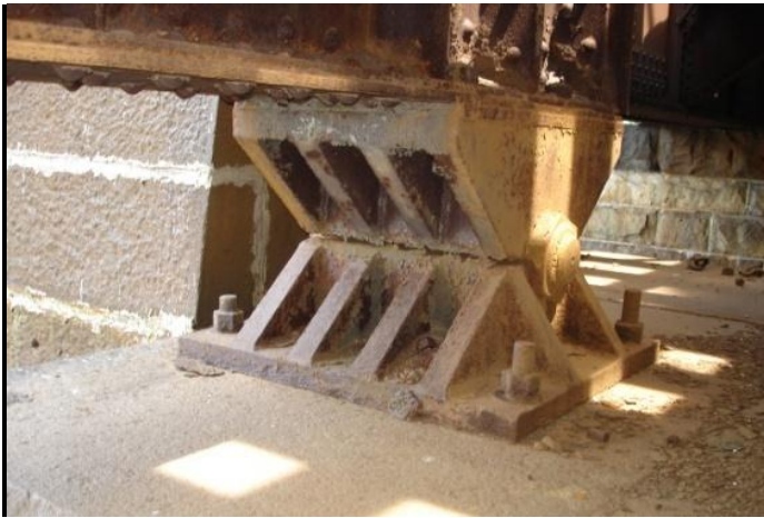
Figure 6.2.1g - Fixed pin bearing with bolster
