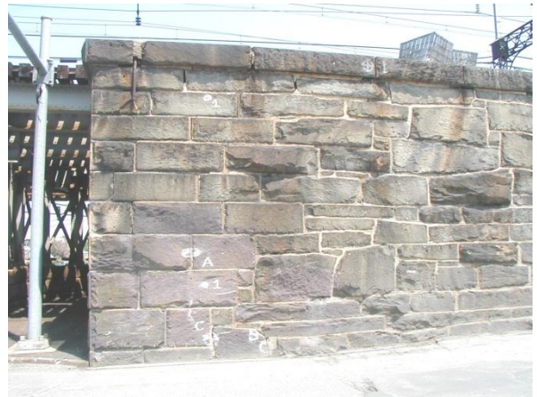
Figure 6.3.2B: Typical Masonry Wingwall
