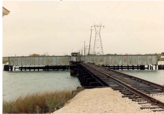
Figure 6.2.6.1d Swing span – girder open position
