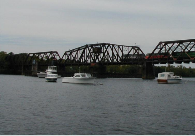
Figure 6.2.6.1a Swing span – truss closed position
