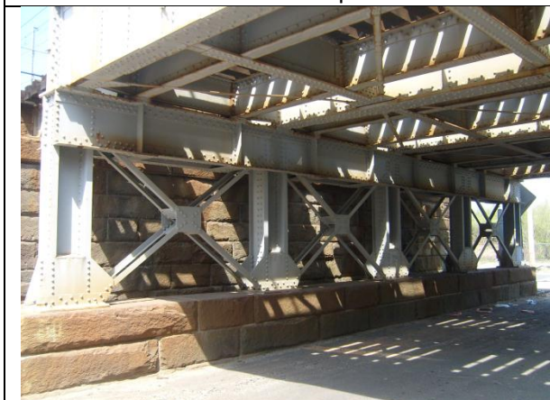
Figure 6.3.3c: Typical steel pier
