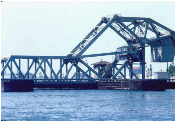
Figure 6.2.6.2a Scherzer type bascule - rolling bascule span truss
