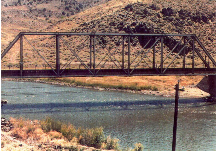
Figure 6.2.5b Pratt Truss – side view
