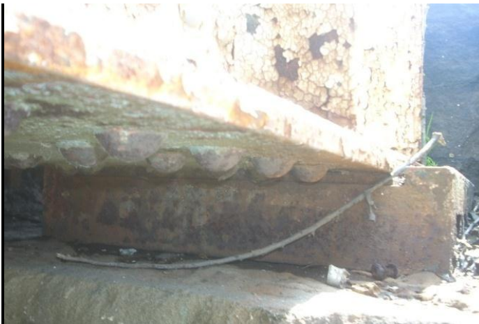
Figure 6.2.1k - Expansion sliding plate bearing
