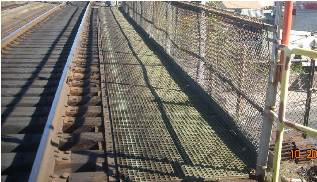
Figure 6.1.6a: Fiberglass Grate sidewalk
