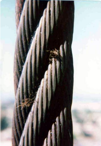
Figure 6.2.6.3n Counterweight ropes - fiber core being expelled
