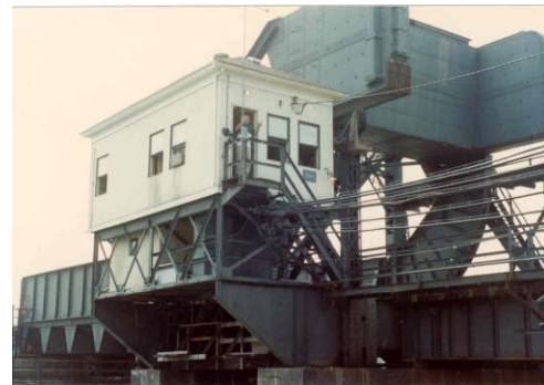
Figure 6.2.6.4b House - adjacent to bridge
