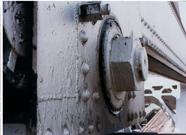
Figure 6.2.6.2p Strauss type bascule - operating strut with rack operating strut guide
