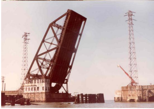
Figure 6.2.6.2a Scherzer type bascule - rolling bascule span truss
