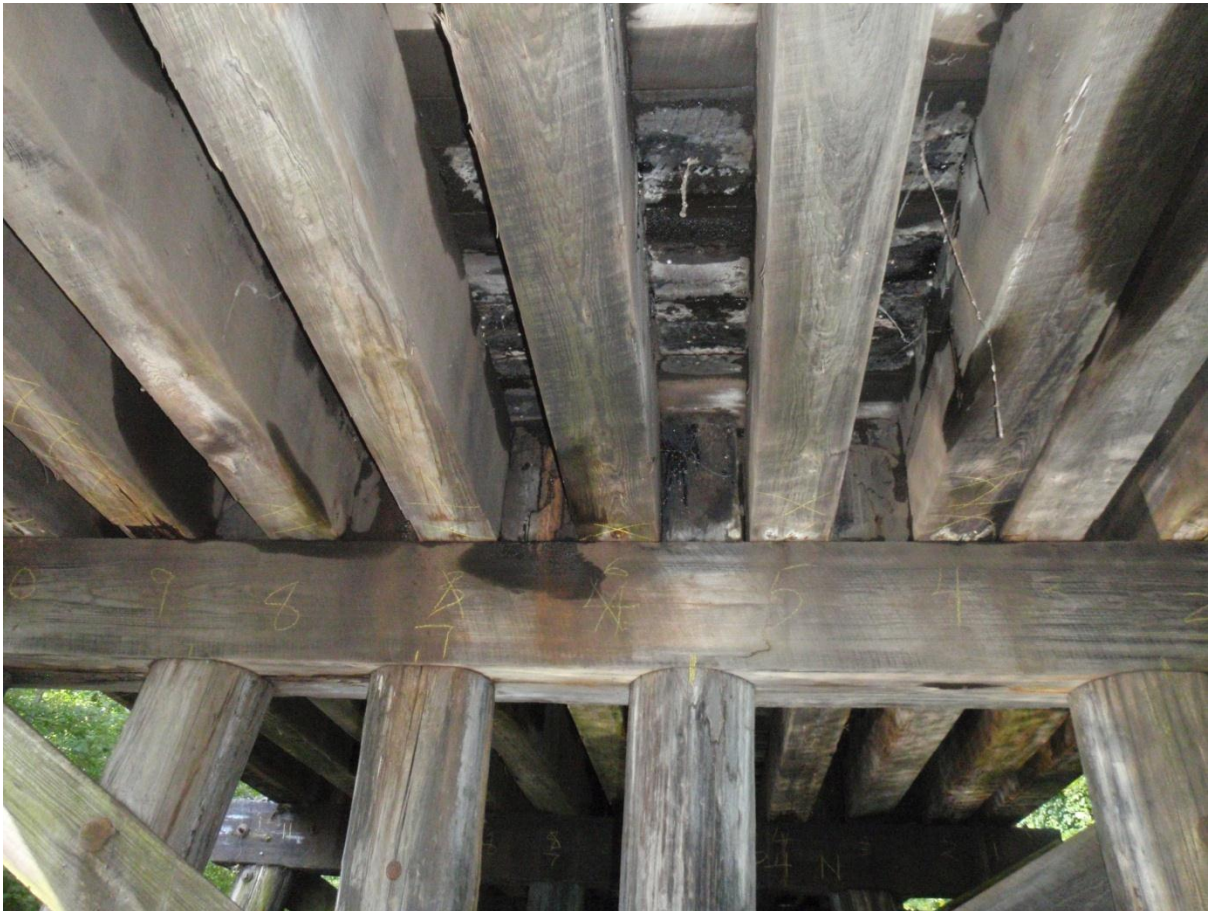
Figure 6.1.3.1b: Underside of a Timber Ballasted Deck
