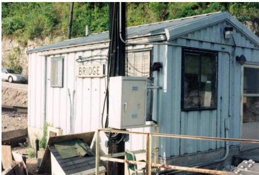
Figure 6.2.6.4a Metal building on shore
