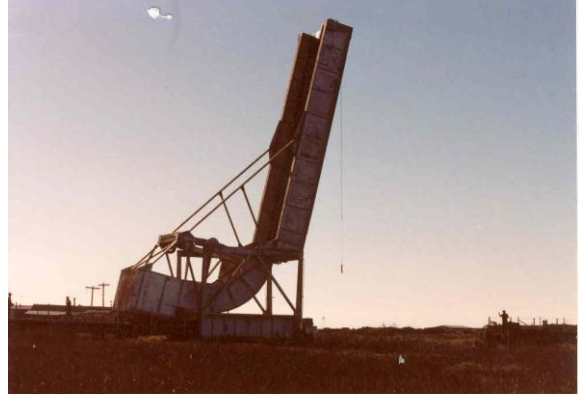
Figure 6.2.6.2b Scherzer type bascule - rolling bascule span girder
