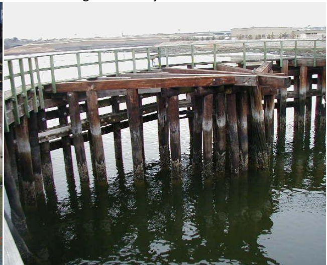
Figure 6.2.6.9l Timber fendering dolphin
