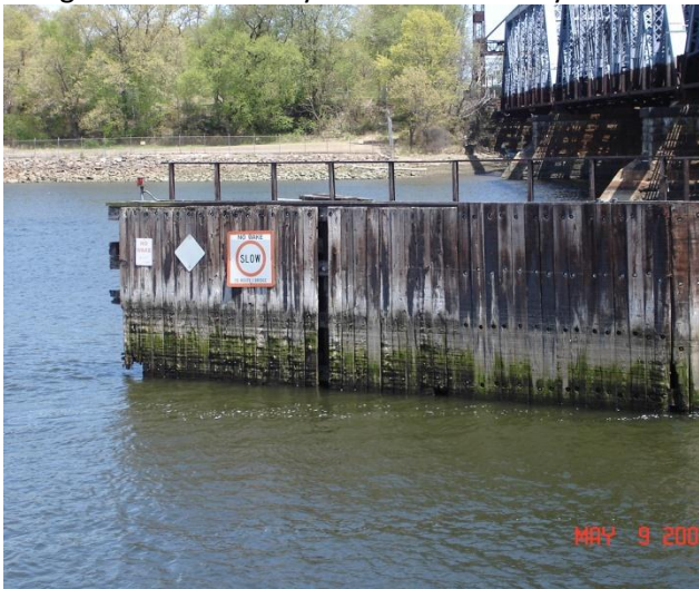
Figure 6.2.6.9k Typical fender system
