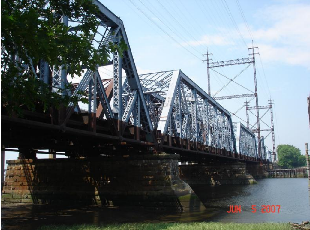
Figure 6.2.4b – Through Truss Bridge.
