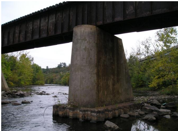
Figure 6.3.1a: Concrete Pier with sheet piling cofferdam footing
