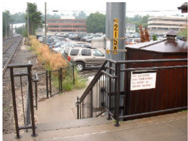
Path to Parking Lot at South End of Platform
