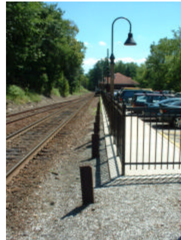
Fence, Walk and Post Mounted Light Next to Track
