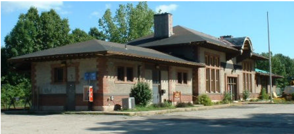
Old Train Station being rehabilitated by the Naugatuck Historical Society
