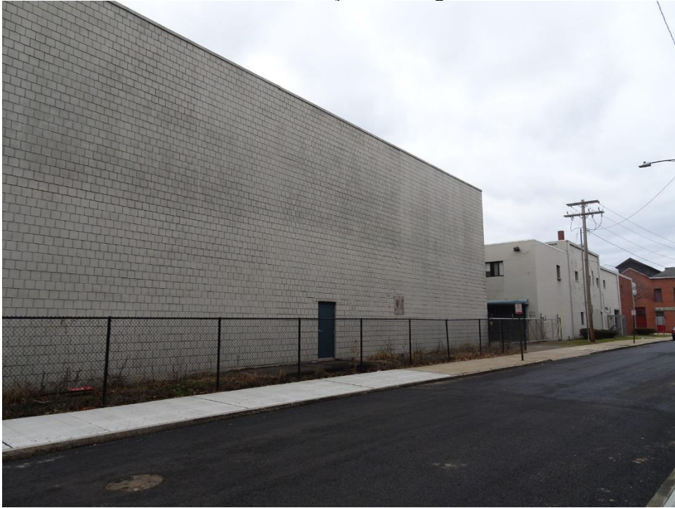
Wallace Street façade looking north
