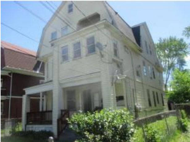
Property Photo Prior to Rehabilitation (Still under construction)
