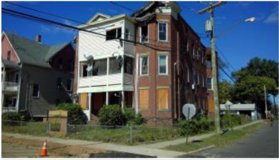
Property Photo Prior to Rehabilitation (Still under construction)
