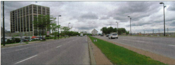
Figure 3. Example of a road with a credible limit of 37 mph (60 km/h)
