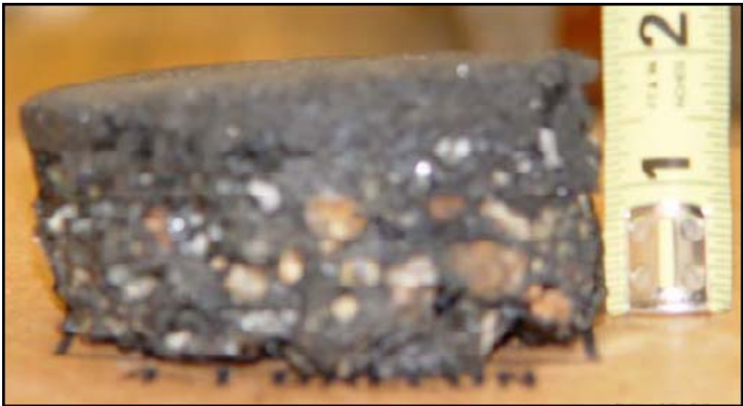
Photo 7 - NH Bridge 102-120 Cores Milton, NH (Not All Cores Shown)
