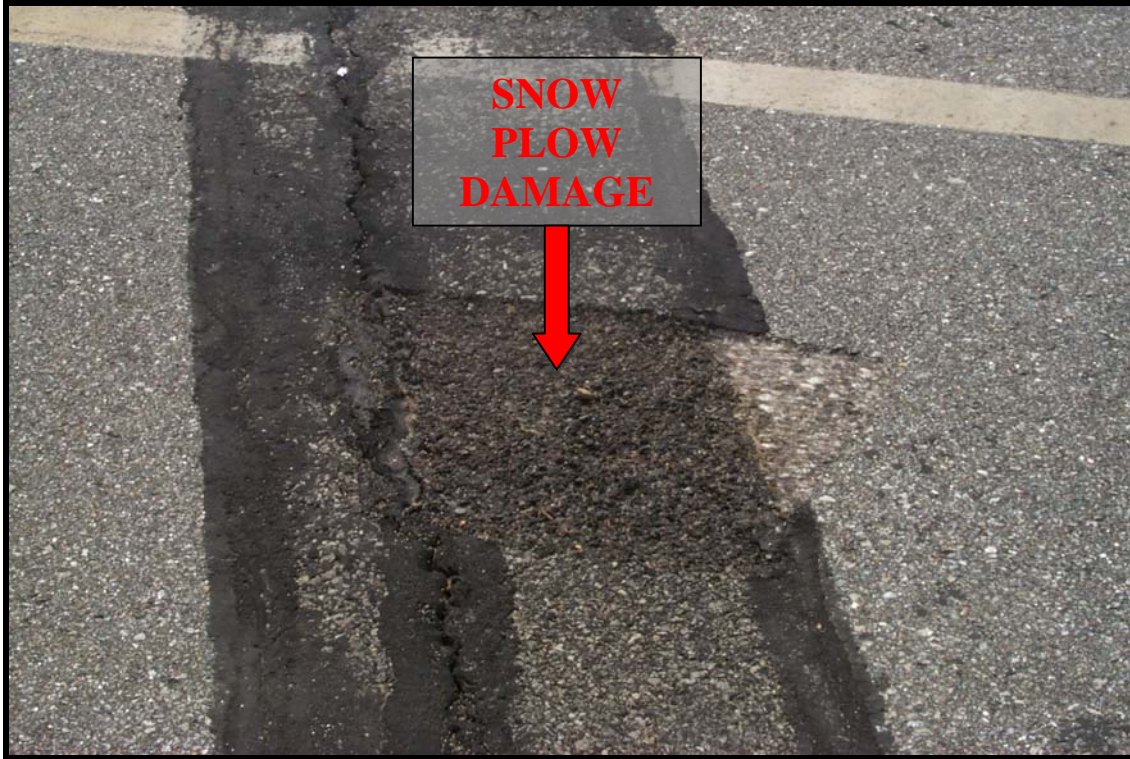
Picture #26: Snowplow damage on bridge #123/173 NH Route 27 over NH Route 101 Hampton, NH
