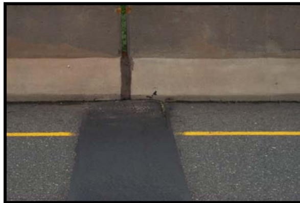
Picture #27: Parapet Detail on Bridge#03313 I-84 TR over 815 New Britain, CT
