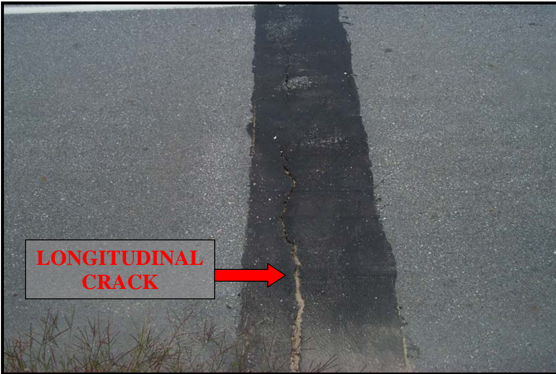
Picture #8: Cracking on bridge #088/126 US Route 4 over Suncook River Overflow Epsom, NH
