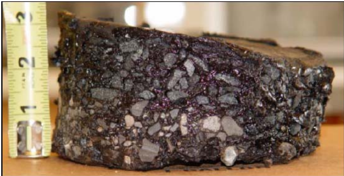
Photo 8 - NH Bridge 109-038 Cores Epping, NH (Not All Cores Shown)
