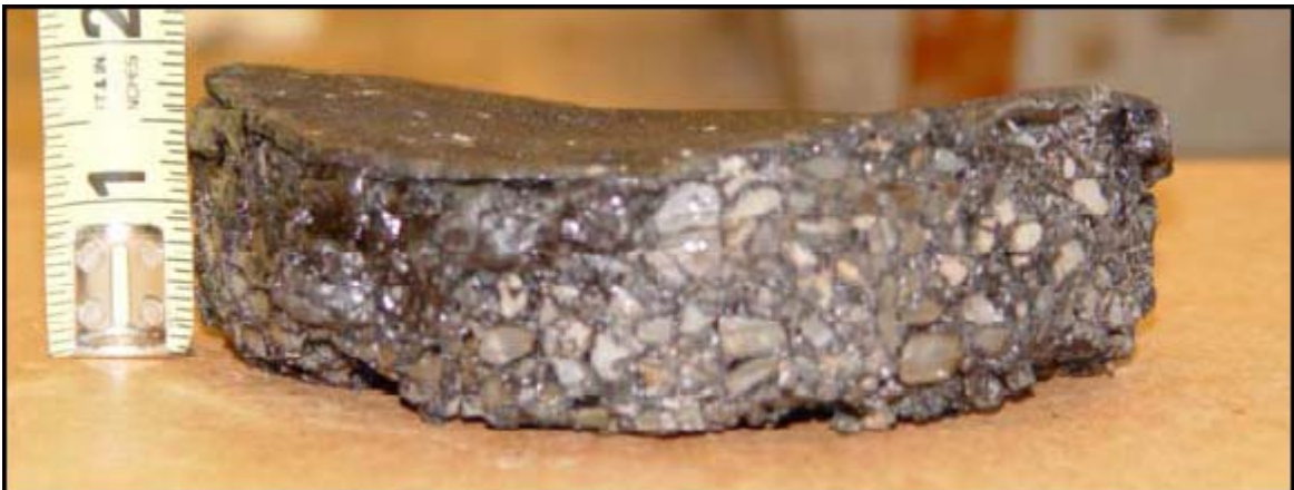
Photo 9 - NH Bridge 123-173 Cores Hampton, NH (Not All Cores Shown)
