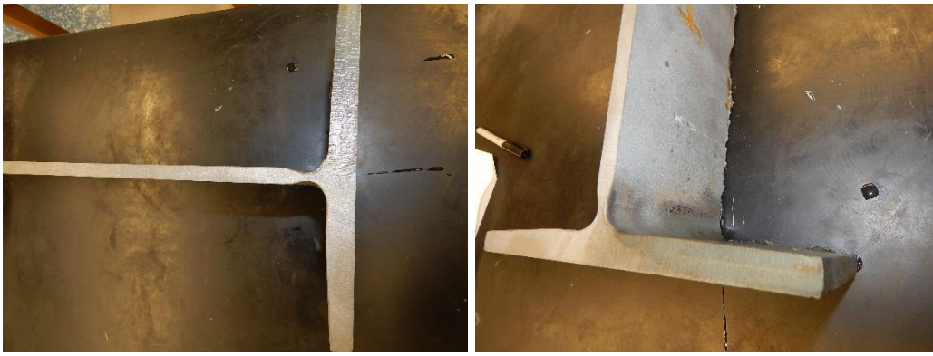
Figure 3.7: Simulation of corrosion damage by sandblasting steel beams
