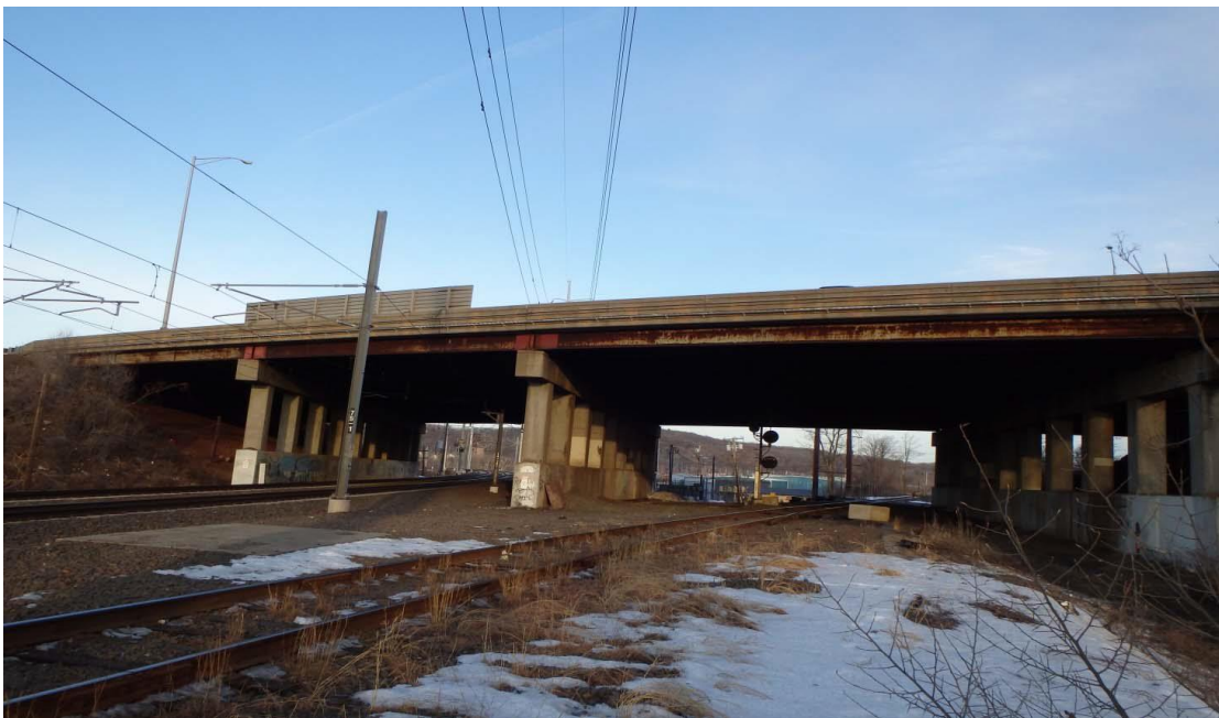
Figure 5.1: Bridge No. 03094 in New Haven, CT, servicing I-91 over Amtrak Railroad
