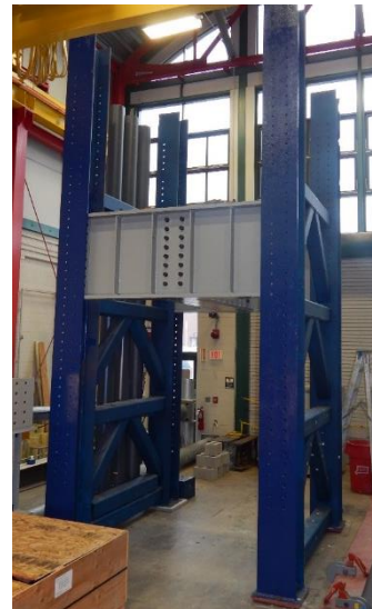
Figure 3.13: Progress of Experimental Test Setup
