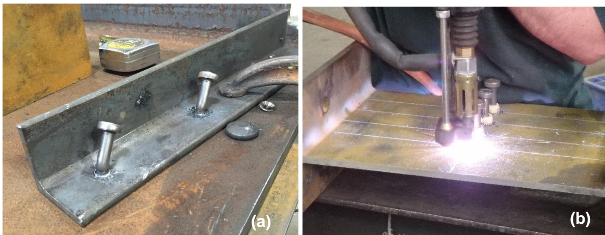
Figure 2.2: (a) bend test on studs; (b) welding using stud gun
