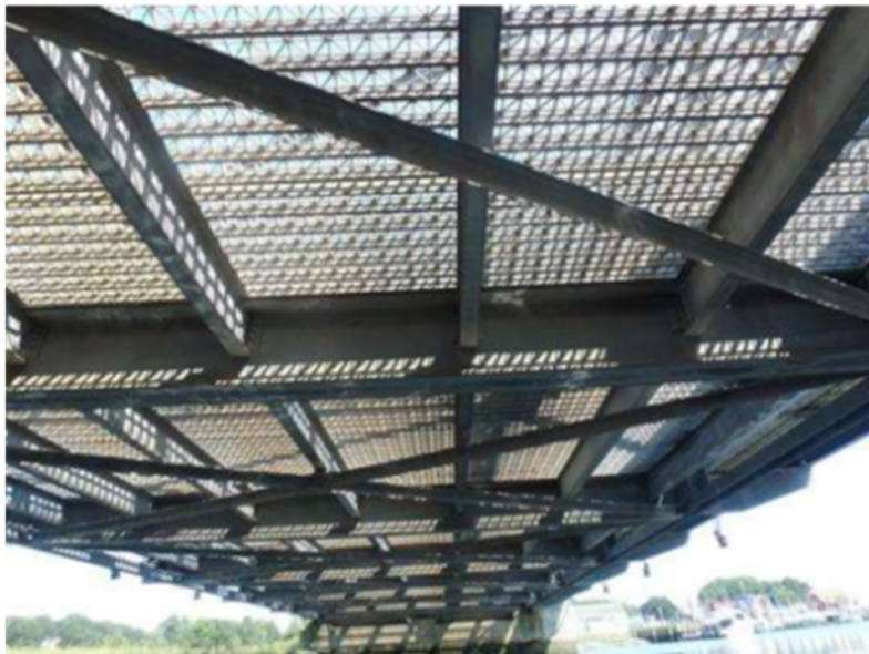
Underside of Steel Grid Deck and Framing Condition- Looking North
