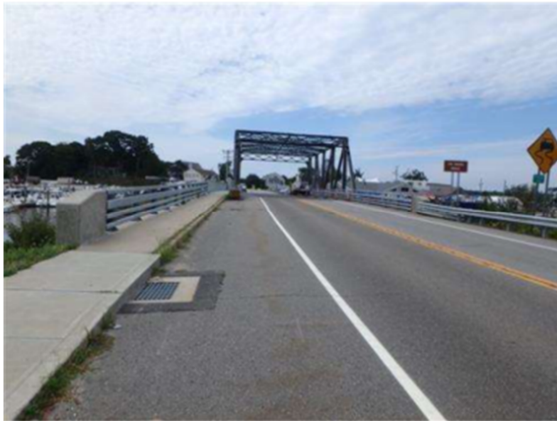
East Approach- looking West
