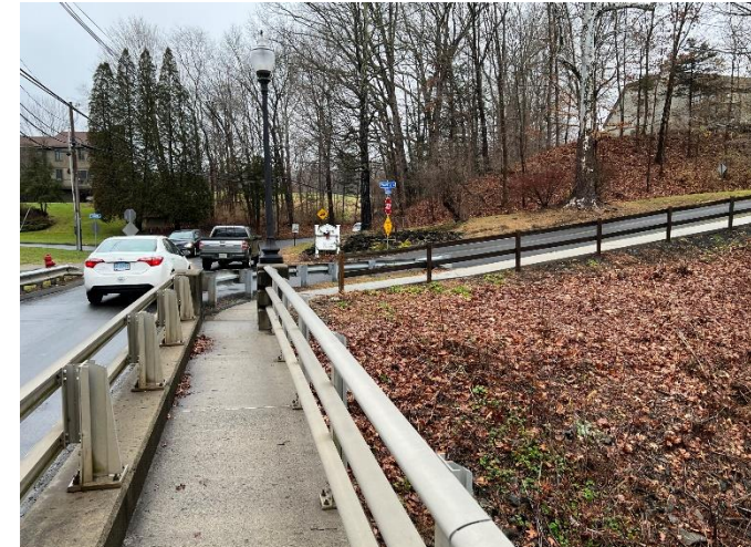
Bridge Sidewalk Condition
