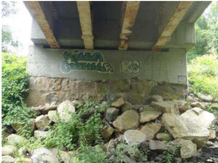
Abutment 1 (West Abutment)
