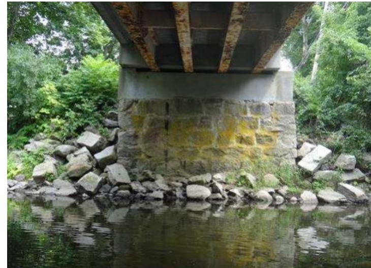
Abutment 2 (East Abutment)
