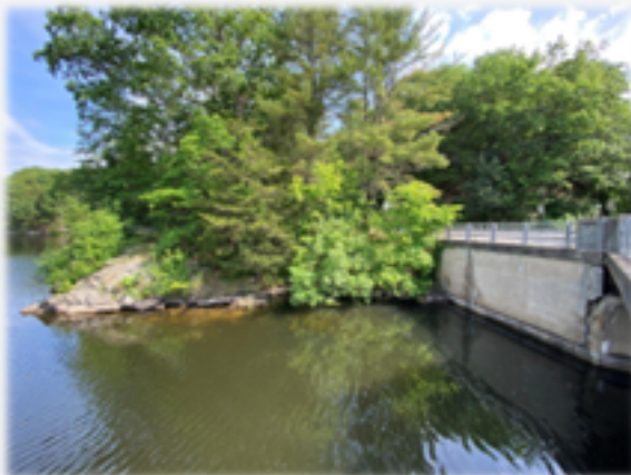
Northwest embankment and exposed ledge
