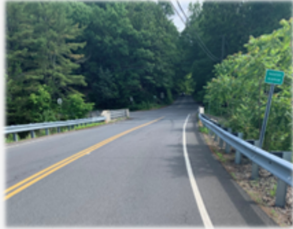
Bridge from South Approach
