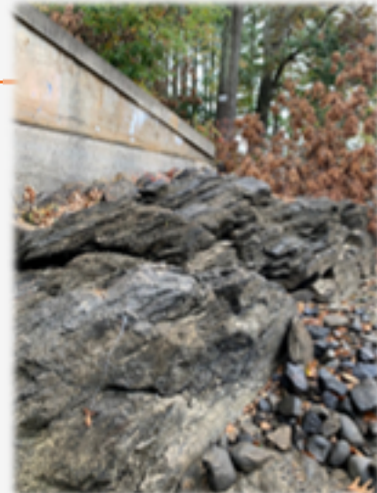
Northeast embankment and exposed ledge
