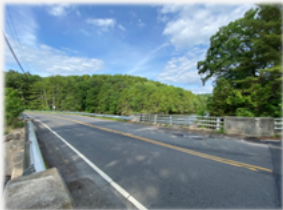
Bridge from North Approach
