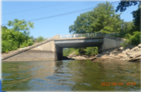
Downstream (East) Elevation
