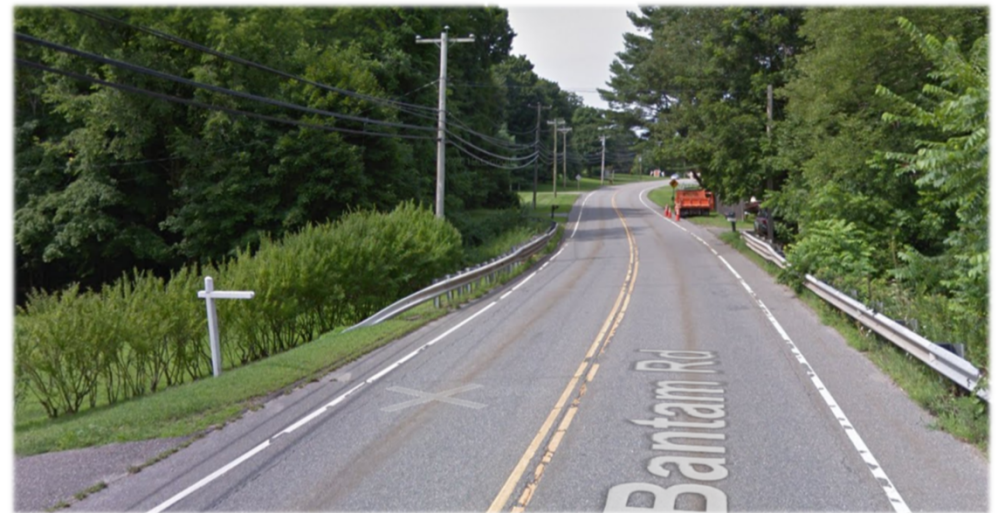
Bridge From East Approach
