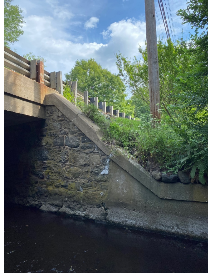
Replacement of Bridge No. 02231 // State Project No. 0073-0194
