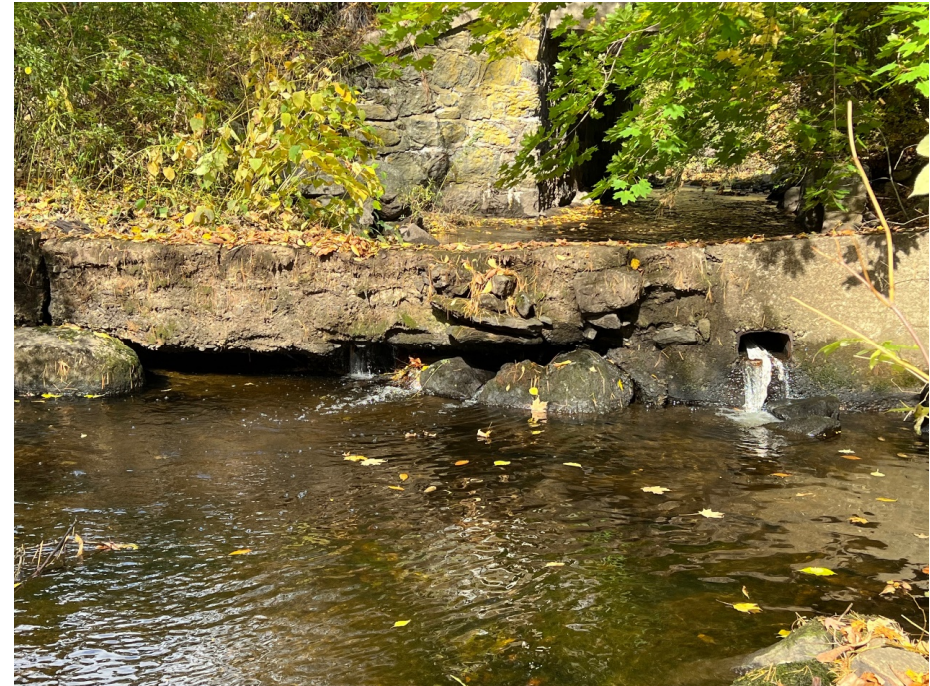
Replacement of Bridge No. 02231 // State Project No. 0073-0194
