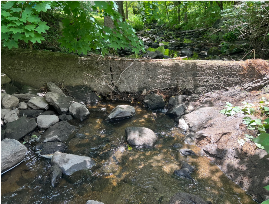
Existing Concrete Dam – Looking Downstream
