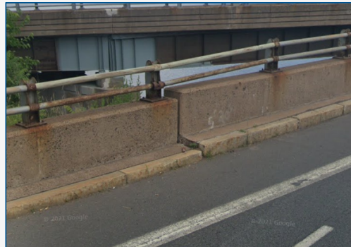
Northwest Retaining Wall
