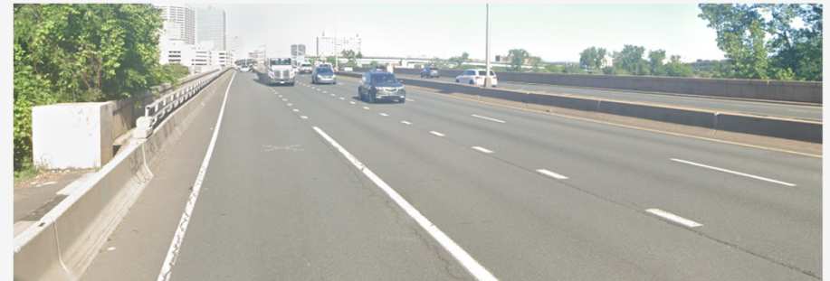
Rehabilitation // Bridge No. 00980A // State Project No. 0063-0734
