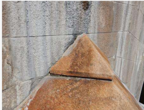
Deteriorated Mortar
