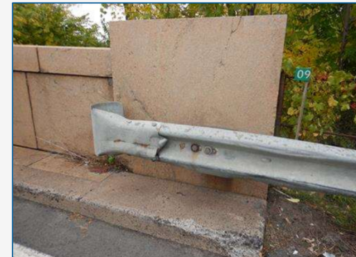
Northeast Approach Guardrail
