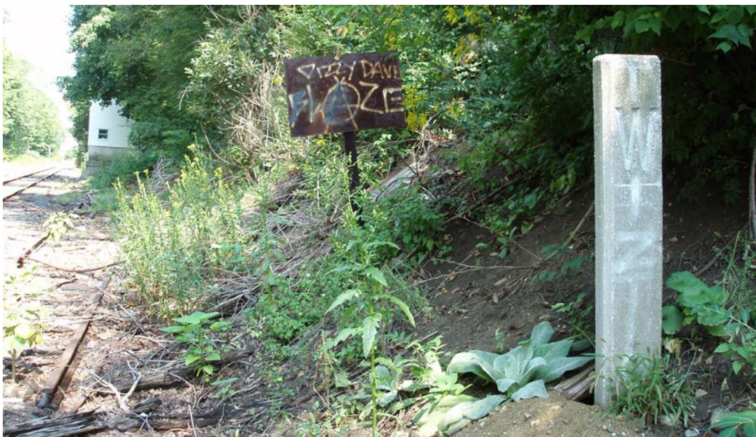
Figure No. 32: North view of concrete whistle post in New Milford, with debossed "W". RR feature #12.
