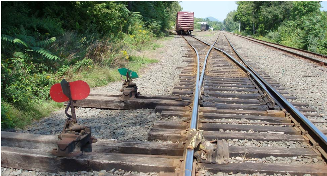
Figure No. 29: Northwest view of manual switching devices at the beginning of a spur for the Kimberly Clark plant in New Milford. Note the green and red signals attached.
