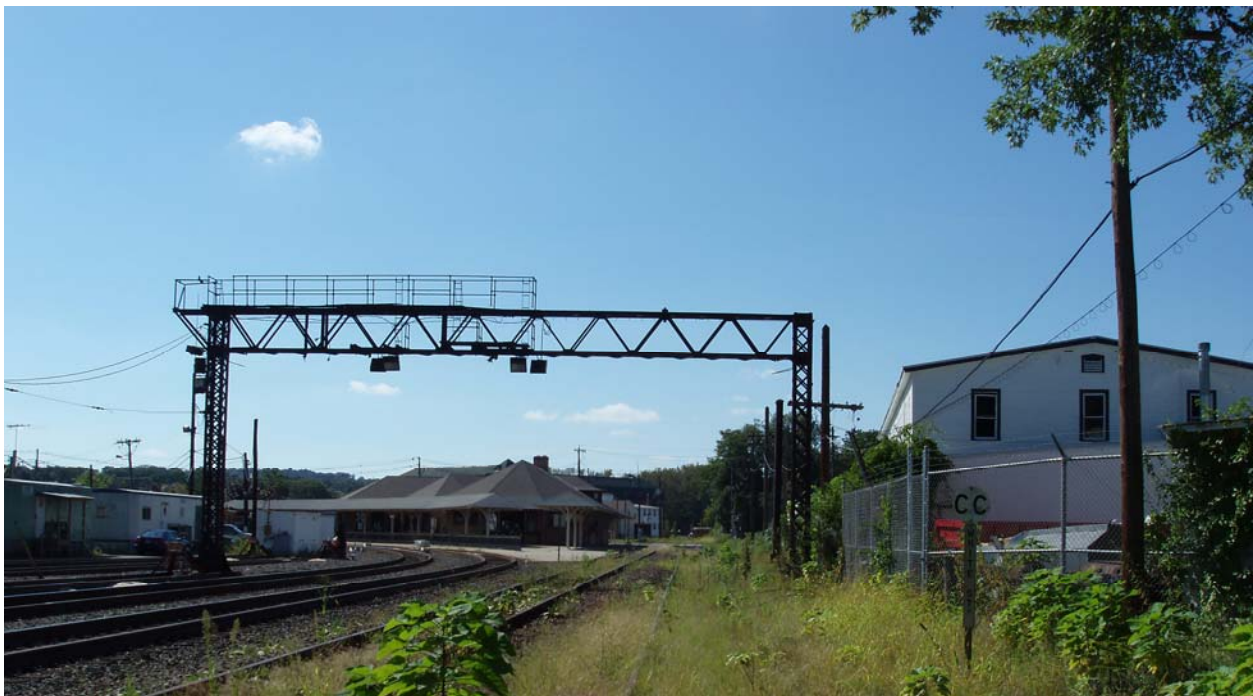
Figure No. 31: West view of catenary structures, associated with the former electrification of the south branch line. Union Station is in the background. RR feature #117.
