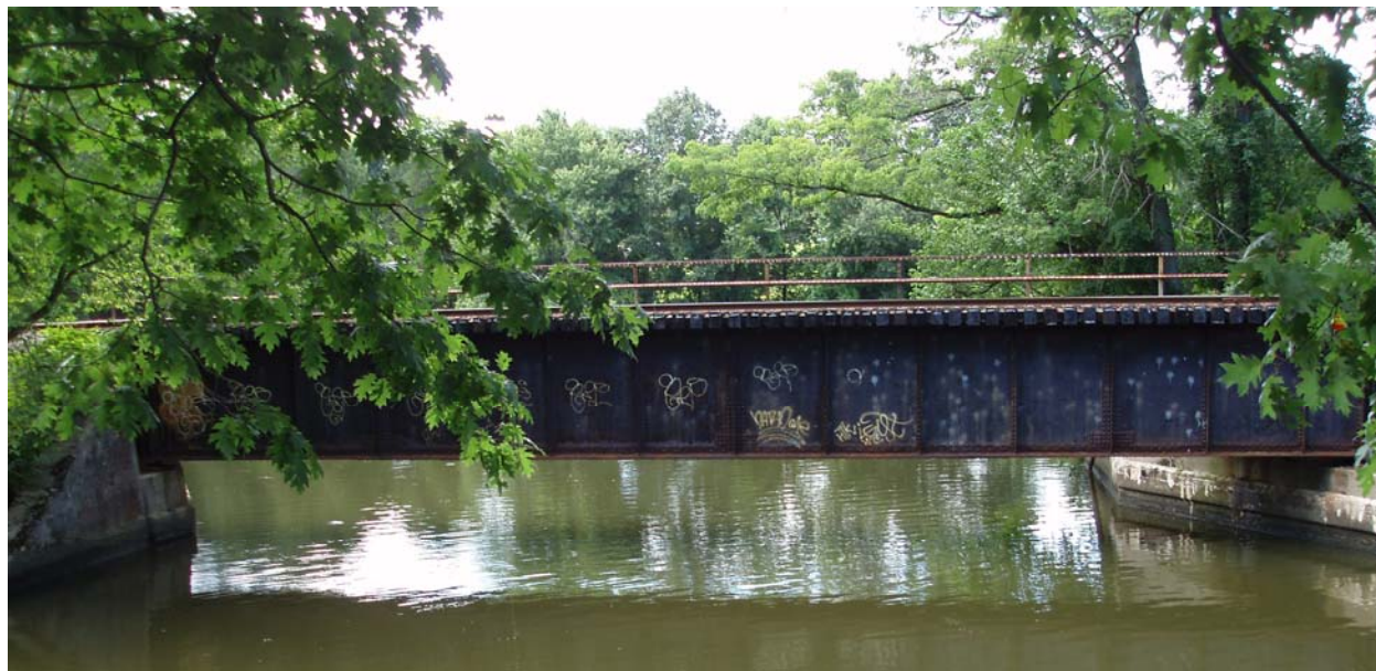
Figure No. 18: West view of the Still River Railroad Bridge which crosses the river in New Milford at the northern end of the Bridgeport Wood Finishing Archaeological Preserve.
