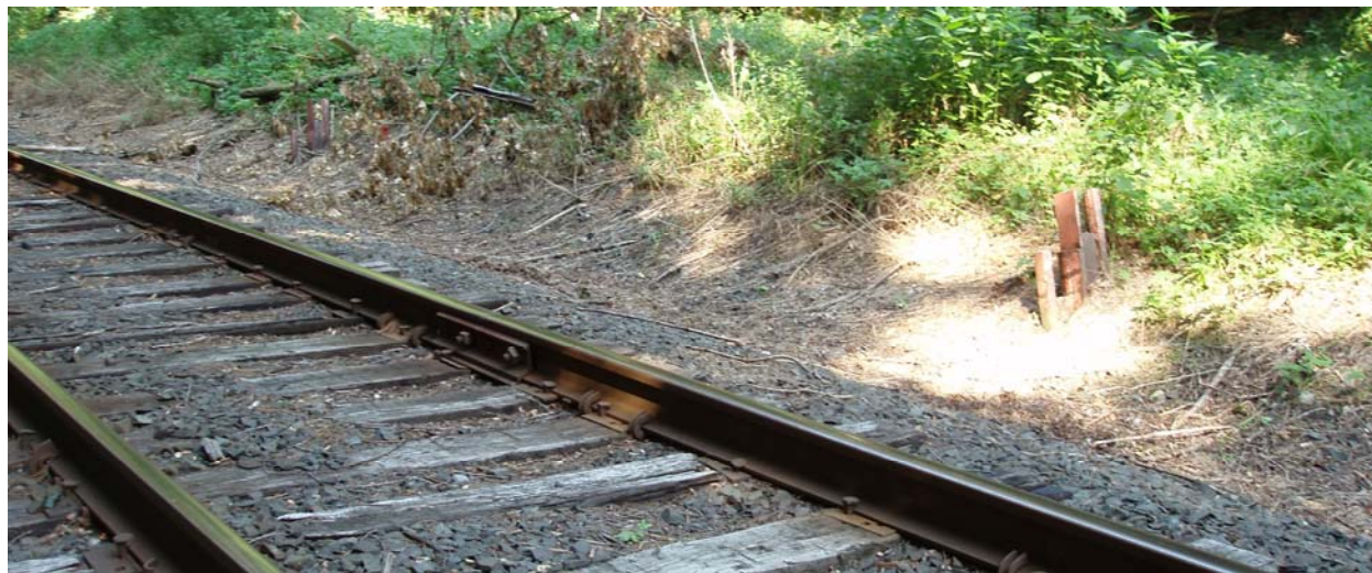
Figure No. 26: Northeast view of custom made rail rack stands on the east side of the tracks, constructed from welded sections of rail, spaced at about 25 feet apart. RR feature #28.
