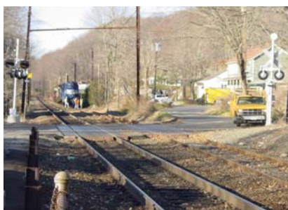
Passing siding on the Branch.
