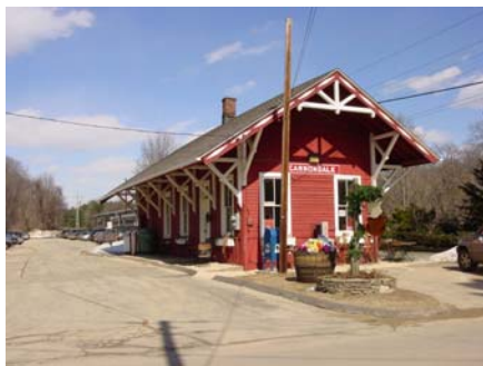
Existing Cannondale Station.
