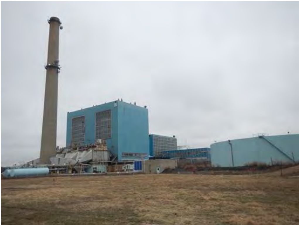
Photograph 12: View from Parcel 5/86/1, looking northwest within the Staging and Storage Area at the power plant. Facing northwest. 3/12/2020.
