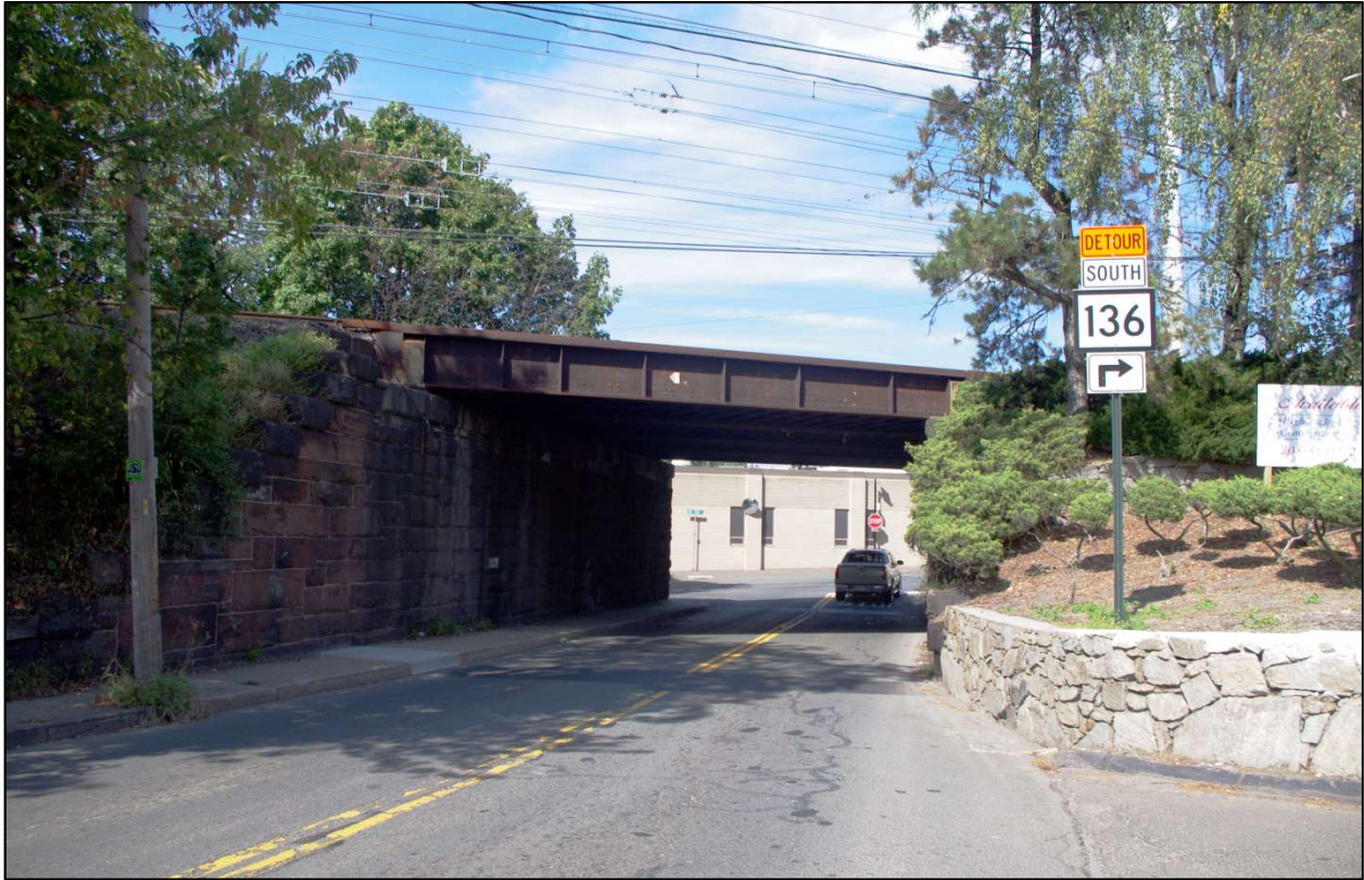
Photograph 1: Fort Point Street Railroad Bridge (1941), south elevation, camera facing north.
