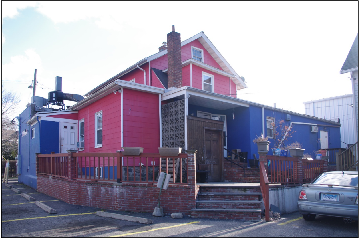
Photograph 7: Rear of house at 21 Fort Point Street, currently in use as a restaurant, camera facing southeast.
