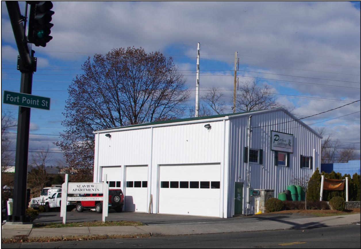
Photograph 12: Commercial garage (2015), 19 Fort Point Street, camera facing northwest.
