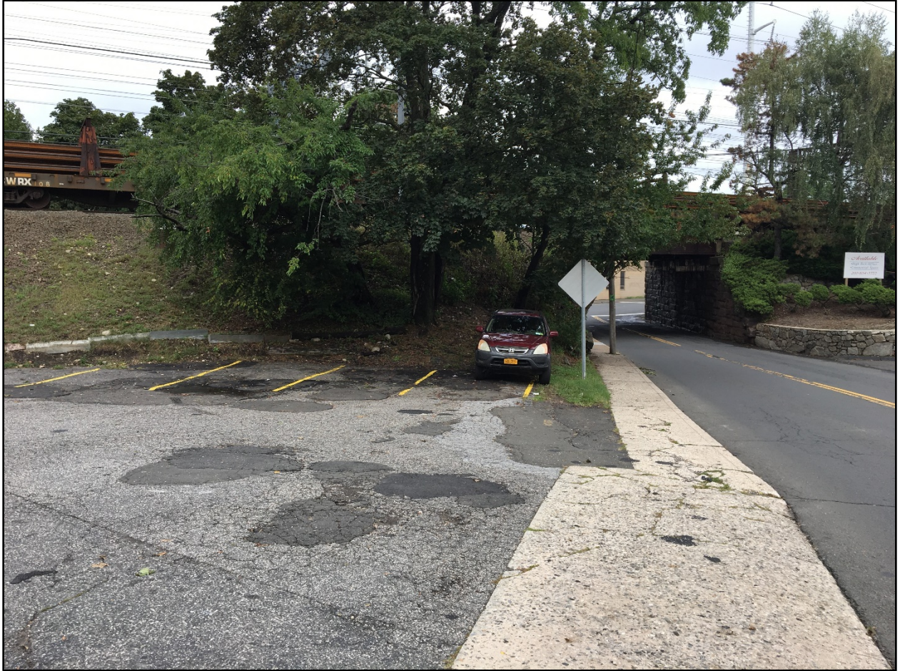
Photograph 1: Existing Fort Point Street Bridge, looking north to area of relocation and where Geoprobe #20 was collected.
