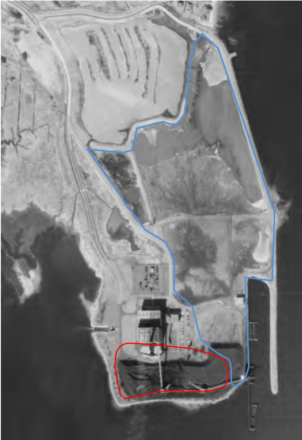
Figure 10: Manresa Island – 1965 Aerial Image. Approximate footprint of the former Manresa Institute identified in red. Note the construction of sea walls and extensive fill (identified in blue) associated with the construction of the CL&P power plant to the northeast, as well as the new power plant and adjoining coal dump themselves.
