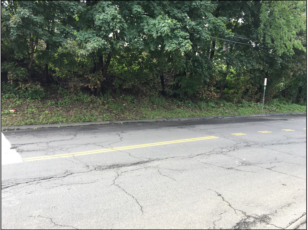
Photograph 3: Fort Point Street relocation area looking southwest.
