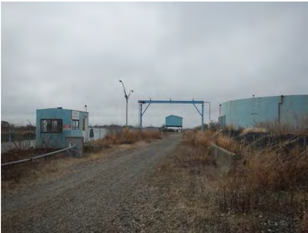
Photograph 6: View from Parcel 5/86/1, looking south within the Staging and Storage Area along the east side of the existing tank farm and west side of the wharf area. Facing south. 3/12/2020.
