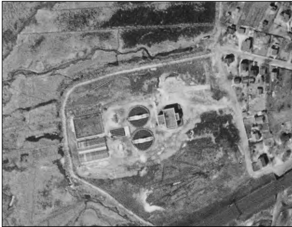
Figure 7: The water treatment plant as shown on the 1934 Fairchild aerial photograph.
