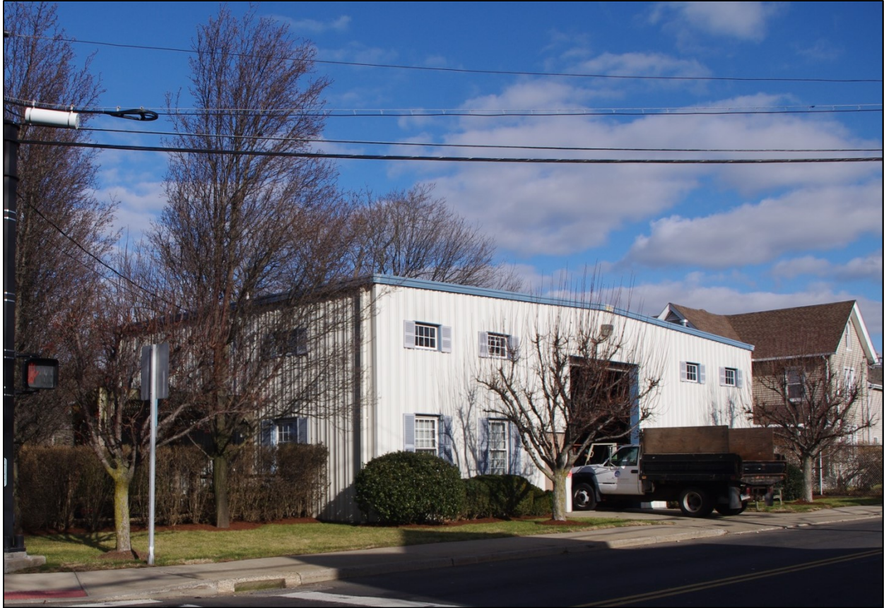
Photograph 14: Commercial garage (2003), 1 Van Zant Street, camera facing east.
