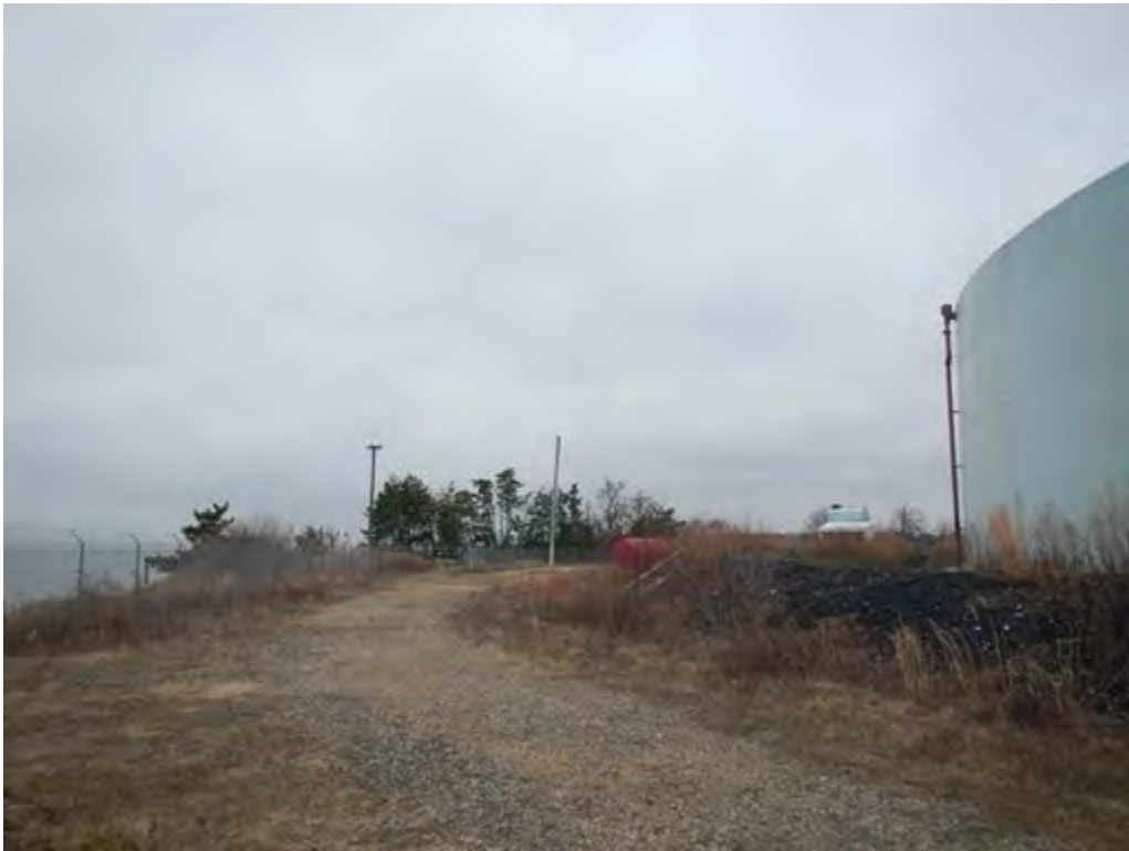
Photograph 8: View from Parcel 5/86/1, looking west within the Staging and Storage Area along the south side of the existing tank farm. Note the gravel surface conditions throughout the area. Facing west. 3/12/2020.
