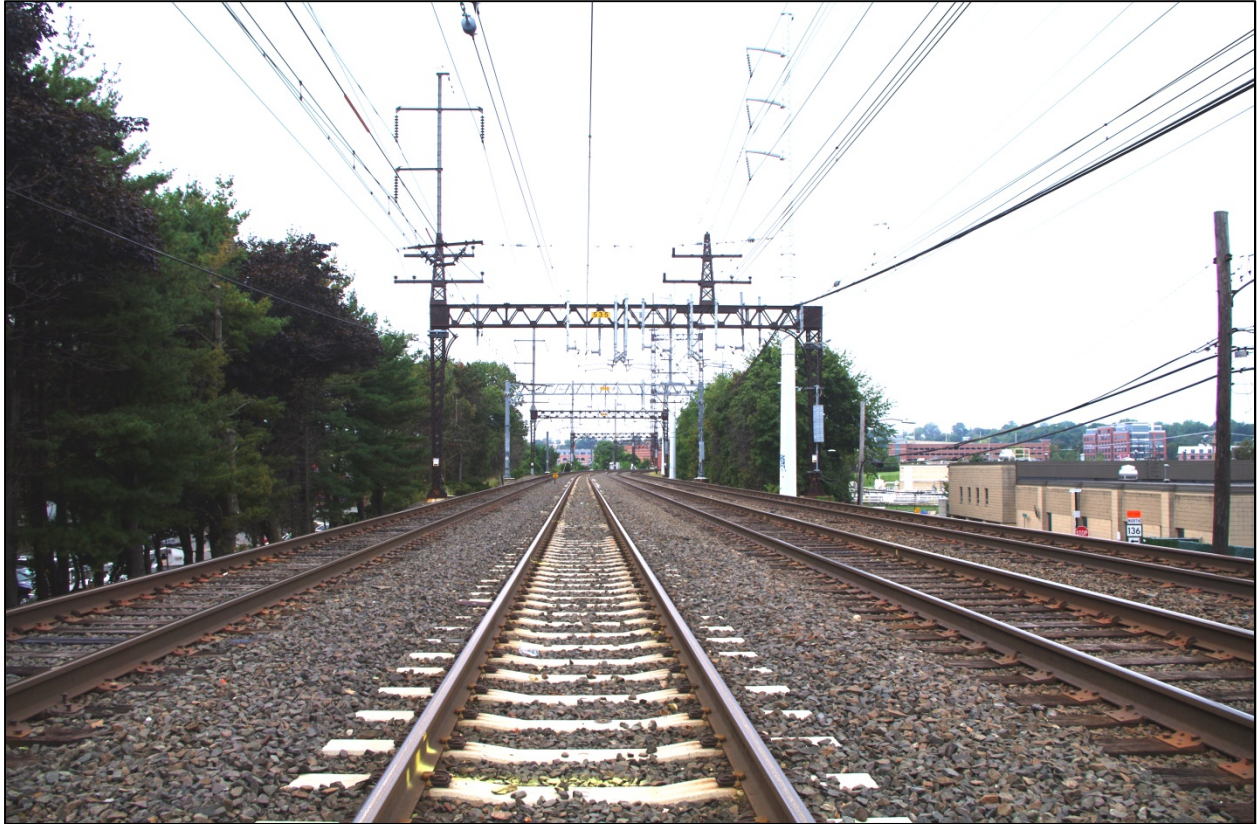
Photograph 3: Track level view of Fort Point Street Bridge, showing historic catenary support structure from the 1914 electrification, camera facing southwest.
