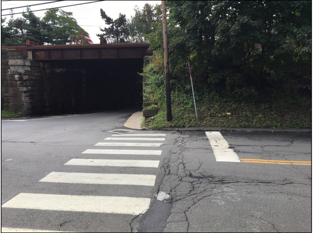
Photograph 2: Existing Fort Point Street Bridge and relocation area looking south.
