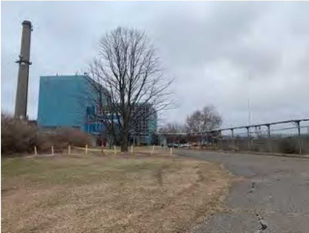
Photograph 1: View from Parcel 5/86/1, looking west within the Staging and Storage Area towards the power plant from the north side of the tank farm. Facing west. 3/12/2020.
