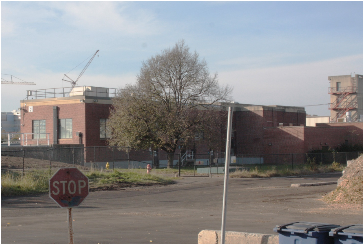
Photograph 10: Norwalk Waste-Water Treatment Plant (1931, with later additions), 60 South Smith Street, camera facing northwest.
