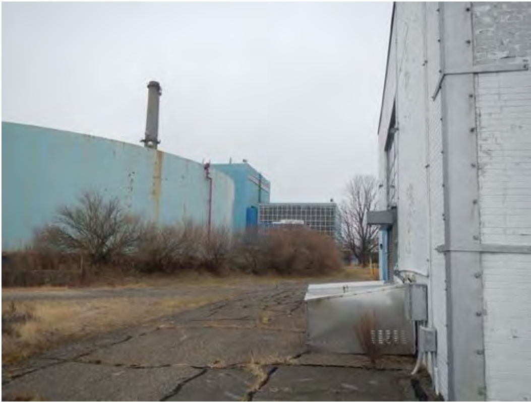
Photograph 5: View from Parcel 5/86/1, looking west within the Staging and Storage Area past the tank farm towards the power plant. Facing west. 3/12/2020.
