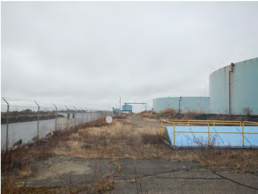
Photograph 2: View from Parcel 5/86/1, looking south within the Staging and Storage Area along the east side of the tank farm and west side of the wharf area. Facing south. 3/12/2020.
