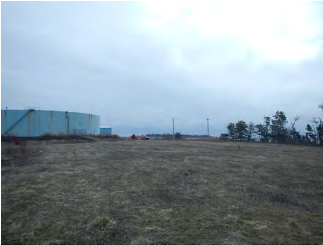
Photograph 13: View from Parcel 5/86/1, looking southeast within the Staging and Storage Area south of the power plant. Facing east. 3/12/2020.
