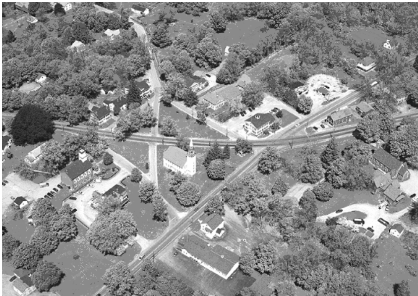
Brooklyn Town Green as it existed before the project (Connecticut Department of Transportation photograph).
