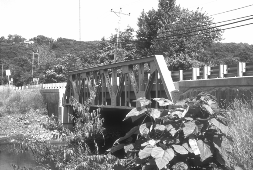
The Route 6 bridge in its original location in Farmington, 1990 (HRC photograph).
