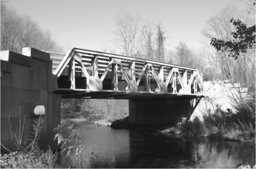
The Route 6 bridge in its new location on Powder Mill Road in Canton.
