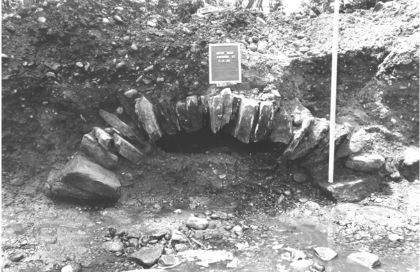
Culvert cross-section, as photo-documented during construction activities (Raber Associates photograph).
