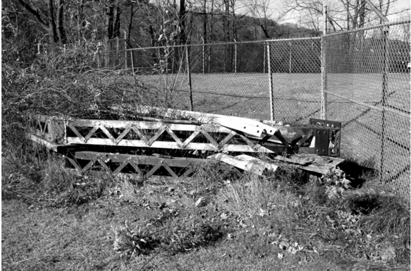
The trusses from the original Powder Mill Road bridge are in storage, awaiting re-erection on a park trail.
