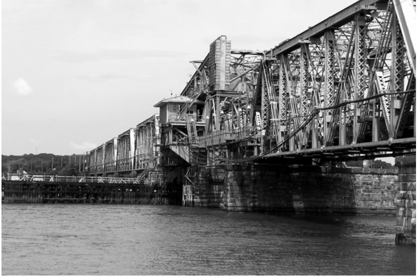
Connecticut River Railroad Bridge, Old Lyme - Old Saybrook, camera facing northwest (HPI photograph).
