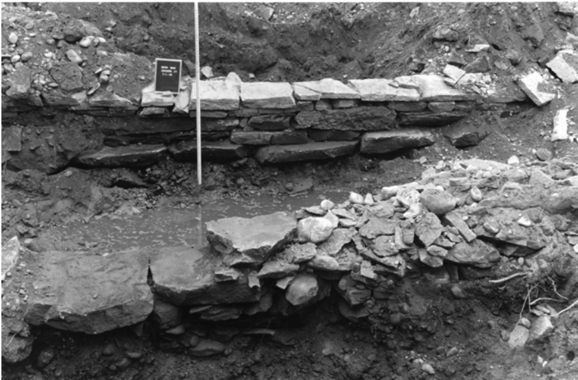
Footings of original Depot Road bridge, as photo-documented during construction activities (Raber Associates photograph).
