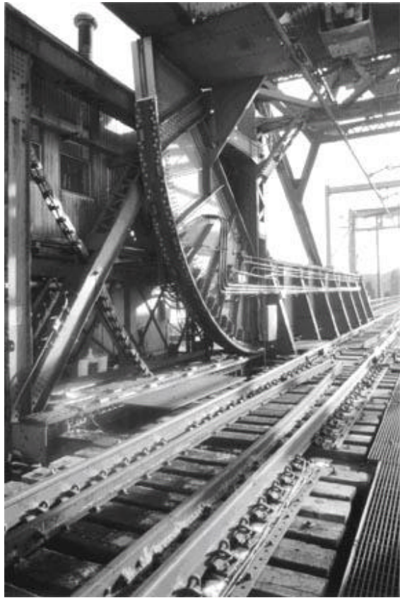
Detail of chain drive and roller segment, Niantic River Railroad Bridge, East Lyme, camera facing southwest (HPI photograph).
