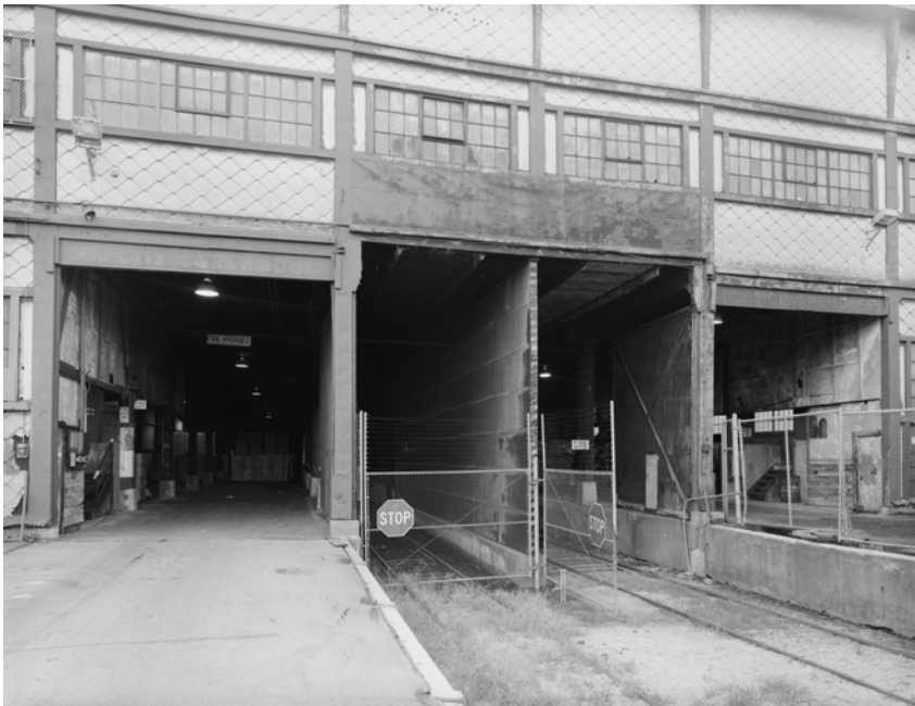
Railroad tracks entered at the north end and ran the whole length of the building. The tracks were depressed below ground level so that the floors of boxcars on the tracks would be at the same level as the warehouse floor (HAER photo by Robert Moore, 1993).
