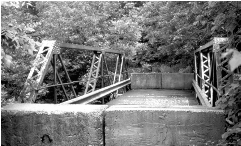
The Powder Mill Road bridge, 1990, closed to traffic (HRC photograph).
