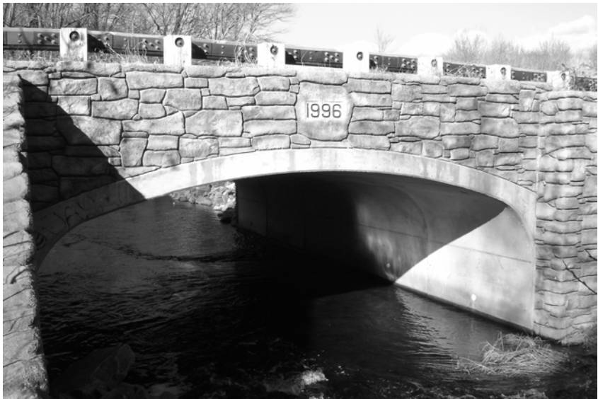
New bridge on Depot Road, completed in 1996.
