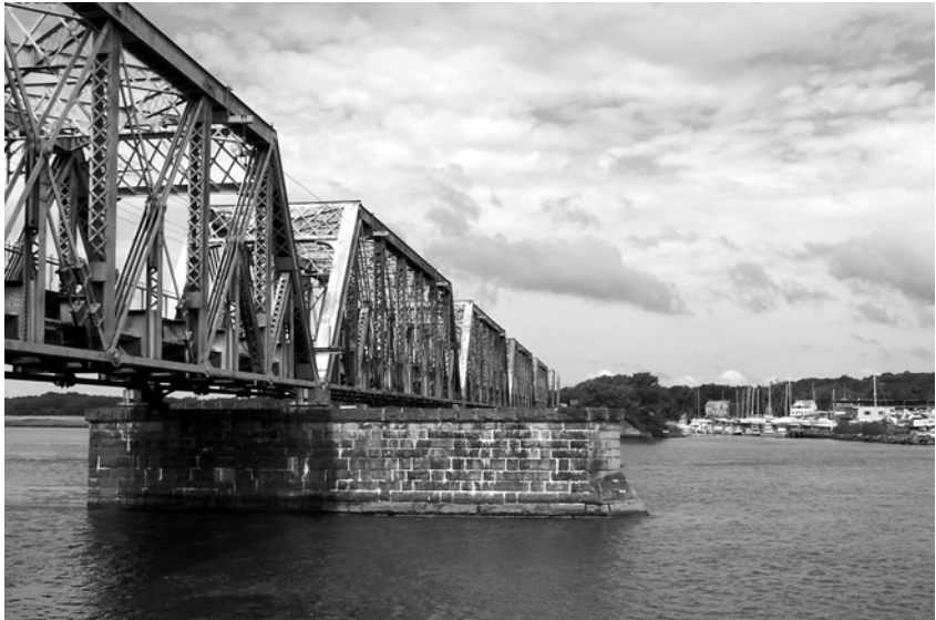
Fixed spans of the Connecticut River Railroad Bridge, Old Lyme - Old Saybrook, camera facing southwest (HPI photograph).
