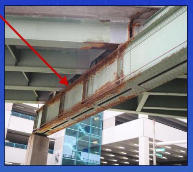
SPALLS WITH EXPOSED REBAR
