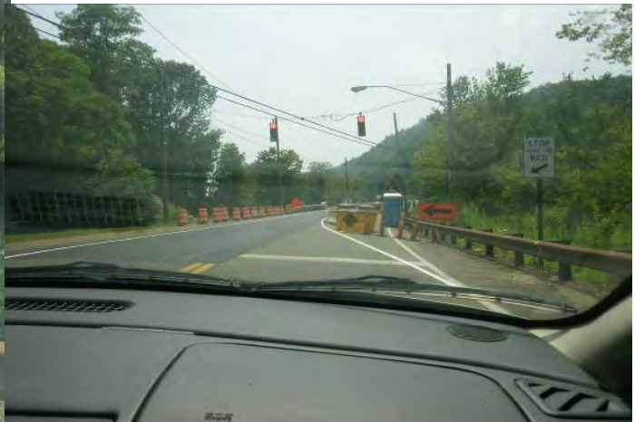
Conflicting pavement markings original was eventually covered with tape.
