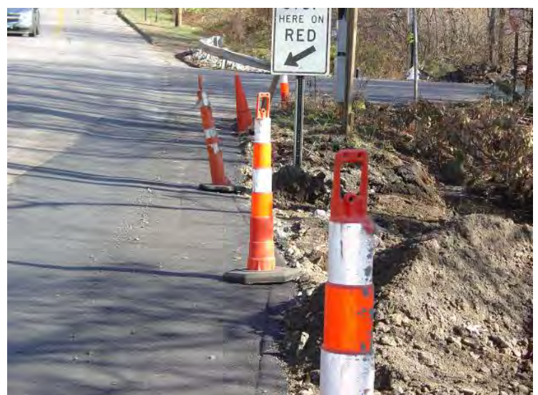
Missing or faded Stop Bar
