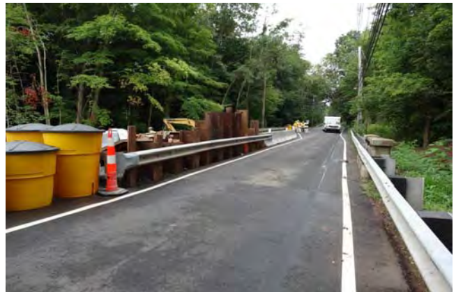
Plan details note the height of temporary earth retaining system shall not extend above the height of the TPCBC.
