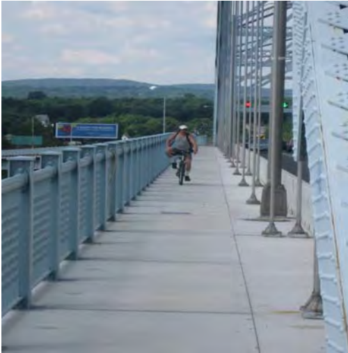
Bicyclist utilizing sidewalk during construction
