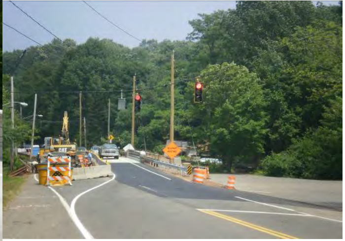
Boat launch in close proximity to stage construction.
