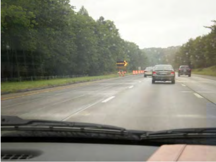
Beginning of Signing Pattern Route 25 Northbound
