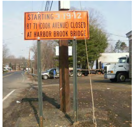
Sign pattern for the road closure at north end of bridge. Barricades were moved to allow for construction equipment access. Barricade stripes should all be sloping downward to the left.
