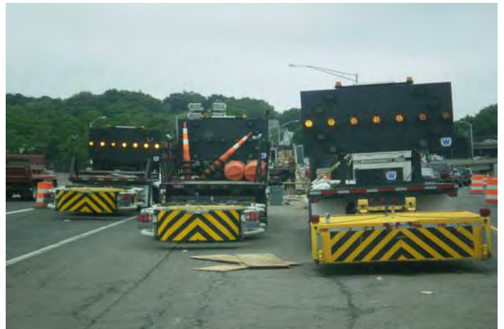
Figure 3: Work Area Protection
