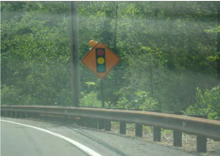
Temporary signalization construction sign high intensity warning light.
