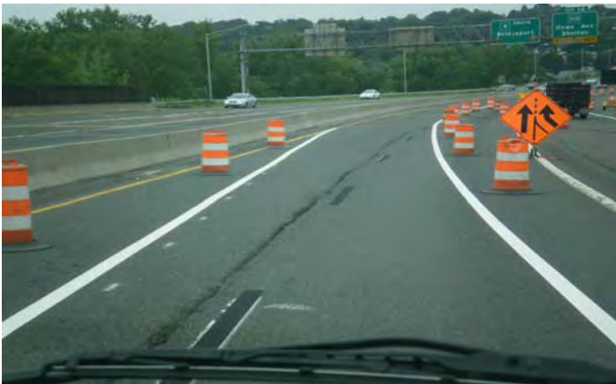
Figure 6: Improper Tape Color
