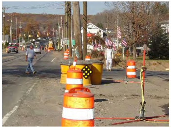
Impact Attenuation System protecting utility poles.
