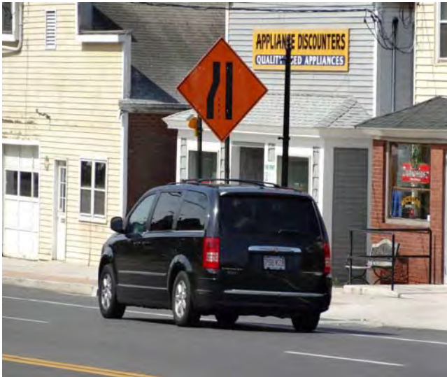
Sign Height for Urban Installation
