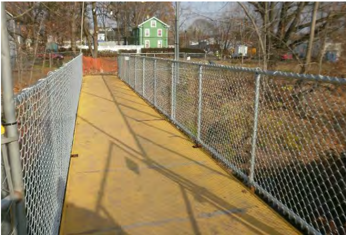
Temporary pedestrian bridge installed around the work zone.
