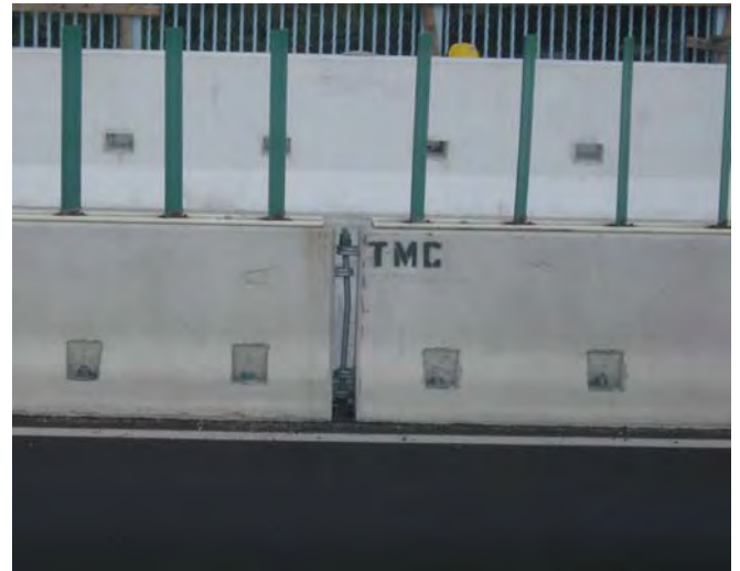
Anchored Barrier Curb with Glare screen
