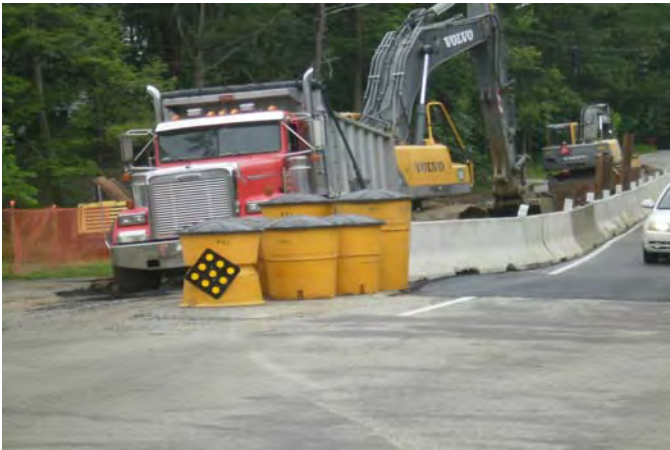
Proper placement of Type A impact attenuation system
