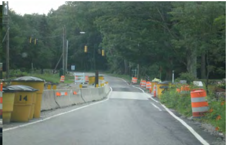
Vegetative Growth obscuring impact attenuation and DE-9 delineator view.
