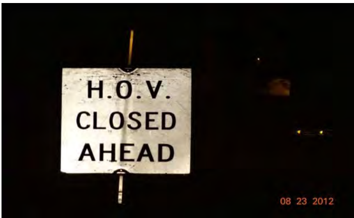
Improper sign type- Using regulatory colors (black and white) versus Construction Sign colors (black and orange). Not included in contract
