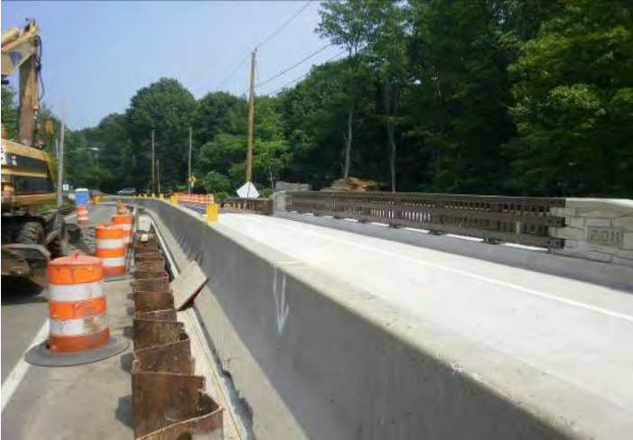
Stage construction with temporary precast concrete barrier curb with delineators.
