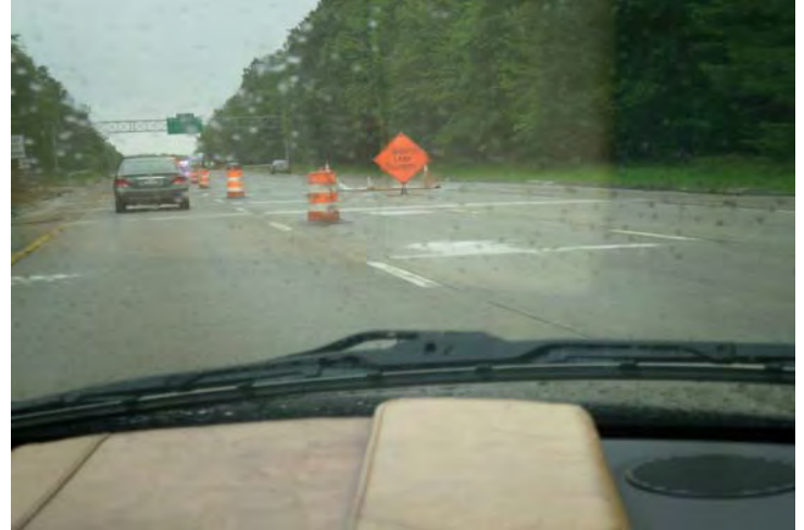
Signs used throughout sign pattern to reinforce lane closure
