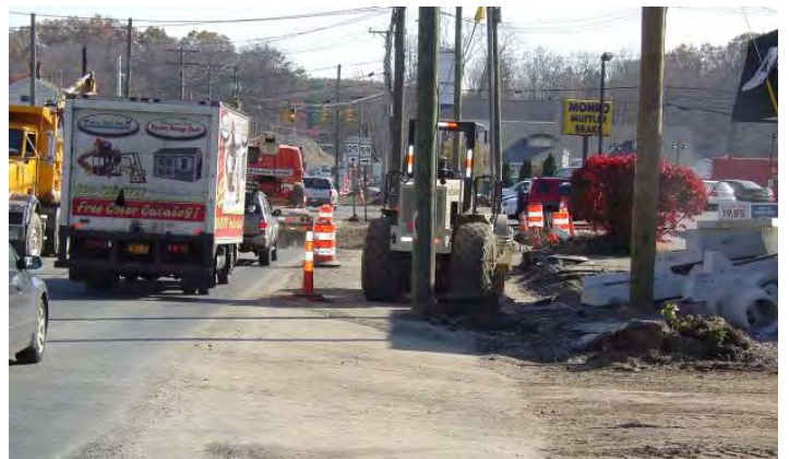
Lunchtime Traffic Queue. Utility pole requiring removal
