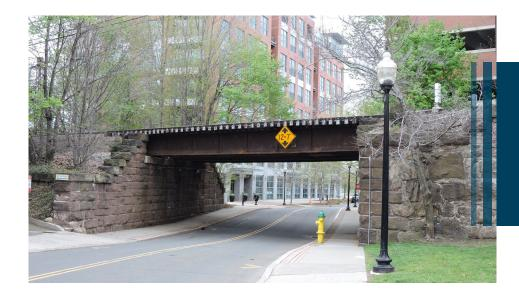
As part of the Danbury Branch Dockyard Project, the superstructure of the rail bridge over Ann Street will be replaced. This includes new weathering steel deck spans, new catenary sytems and abutment wall improvements, which will maintain the 19th century character of the bridge.
