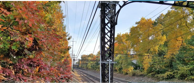
The CP243 Interlocking Project will construct a new four-track interlocking, a powered switch and signal system that allows trains to move from one track to another. The new interlocking is approximately 2,200 feet long, located on the New Haven Line (NHL) between East Norwalk and Westport and approximately 1.5 miles east of the Walk Bridge.
