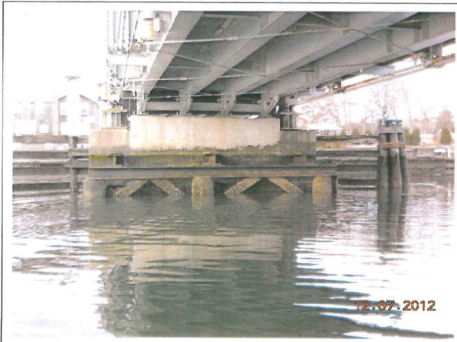
Photo No. 9: Pier No. 2 (East Elevation)
