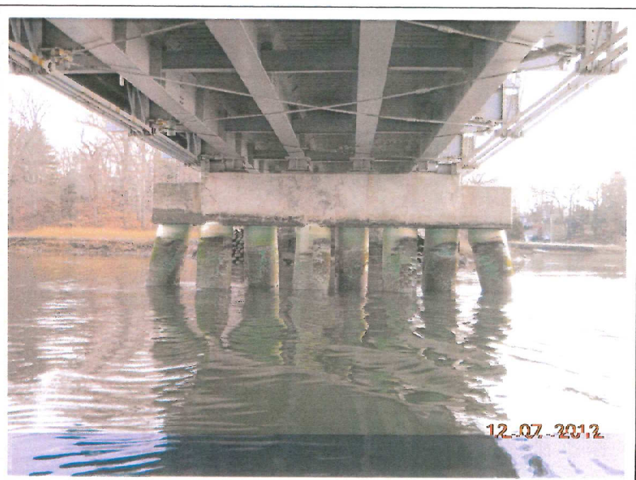
Photo No. 10: Pier No. 3 (West Elevation)
