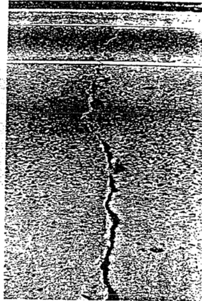
TRANSVERSE CRACKING
