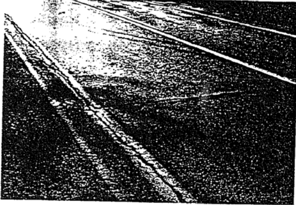
REFLECTIVE CRACKING
