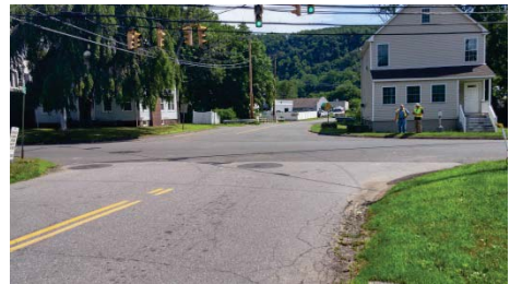
Figure 13. No Pedestrian Facilities
