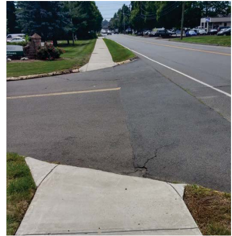
Figure 15. Handicap Ramp at The Willows
