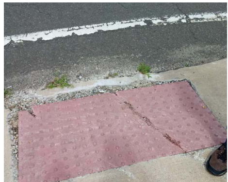
Figure 14. Handicap Ramp at South Corner of Bradley and Amity Road
