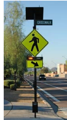
Figure 17: Sample of rectangular flashing pedestrian beacon
