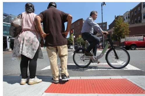
Figure 16: Sample ADA compliant ramps
