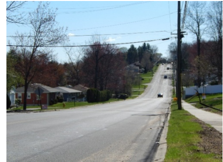
Figure 6: View of Bunker Hill Road corridor facing east
