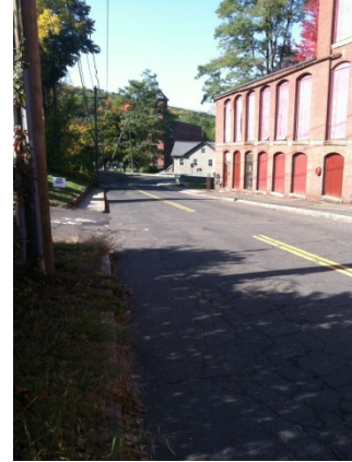
Figure 18. Sidewalk Near the Mill Building.
