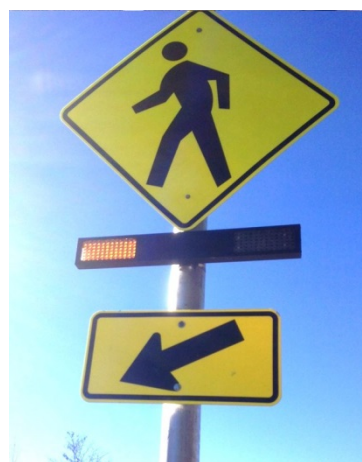
Figure 29. Rectangular Rapid Flashing Beacon
