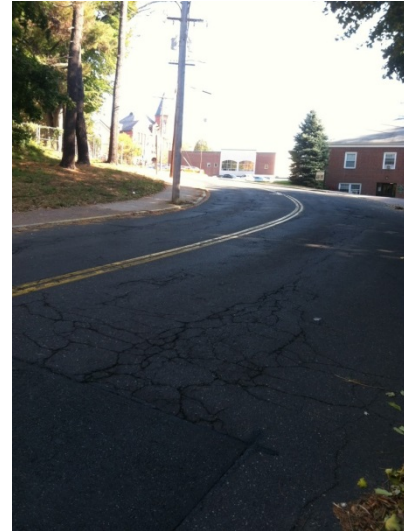
Figure 7. West Main St. looking North
