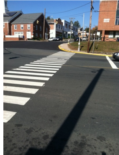
Figure 14. Lack of Sidewalk Ramps at East Main Street/Park Street Intersection
