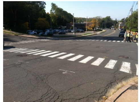
Figure 11. Crosswalks at the Intersection of Brooklyn Street and Court Street
