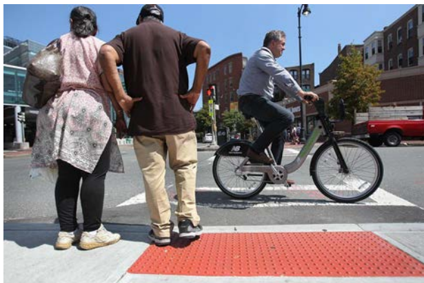
Figure 26. Pedestrian Detectable Warning Strip.
