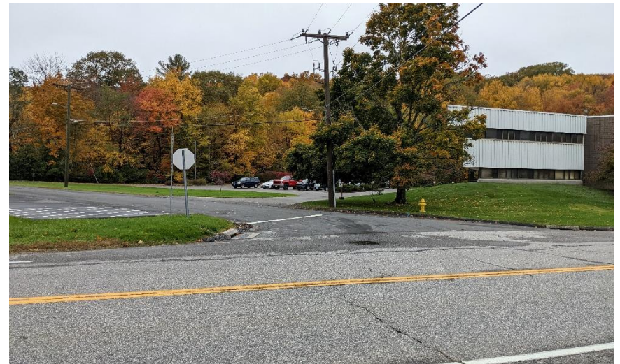
Exhibit 16: The intersection of Route 4 (Goshen Road) and Lovers Lane
