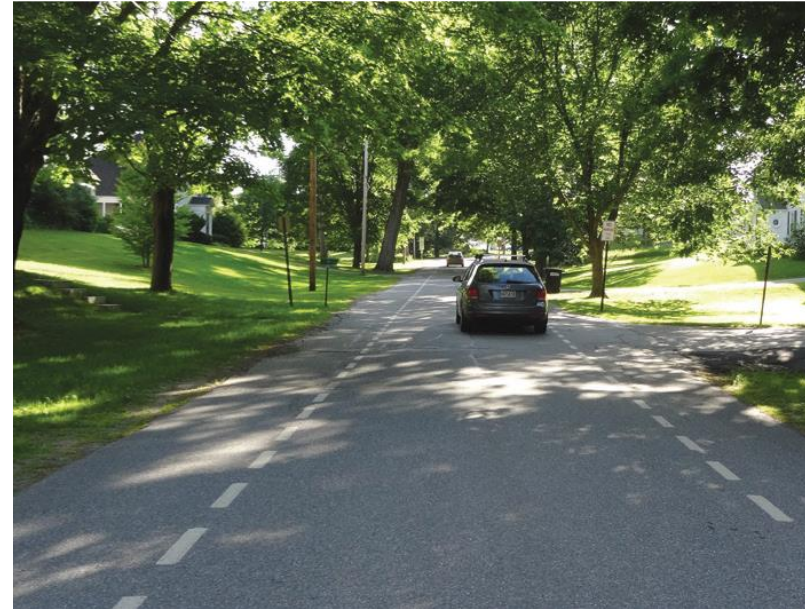
Exhibit 25: Advisory shoulder on a two-way roadway in Hanover, NH (Source: FHWA Small Town and Rural Multimodal Networks Guide)
