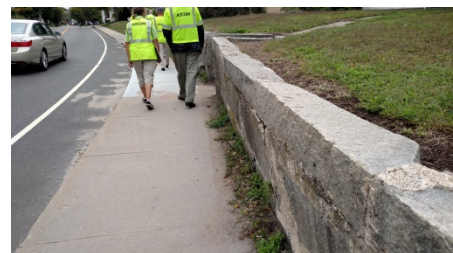
Figure 7. Retaining Wall Against Sidewalk
