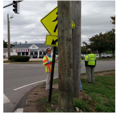
Figure 26. Sign Blocked by Utility Pole
