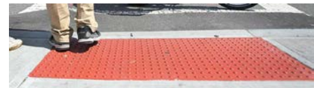
Figure 39. Tactile Warning Strip
