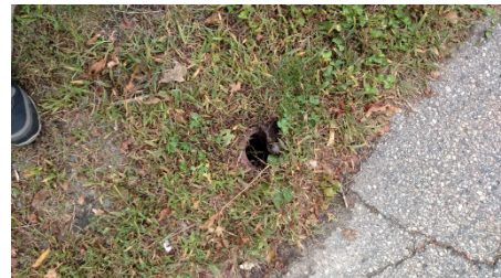
Figure 14. Old Water Valve
