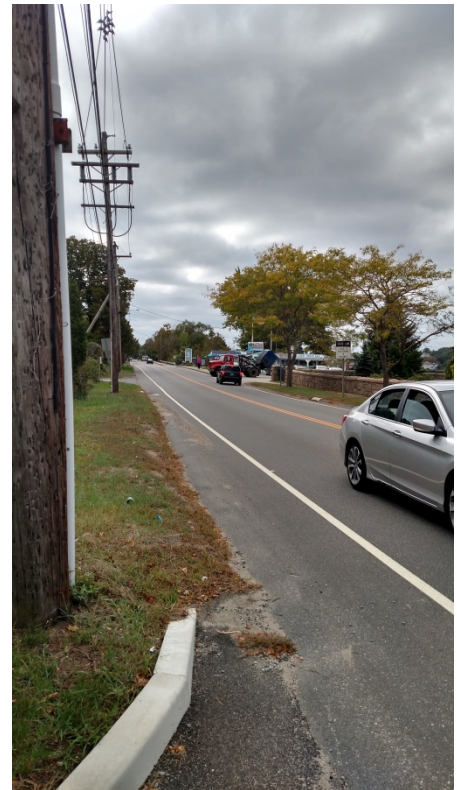
Figure 29. No Sidewalk on the East Side
