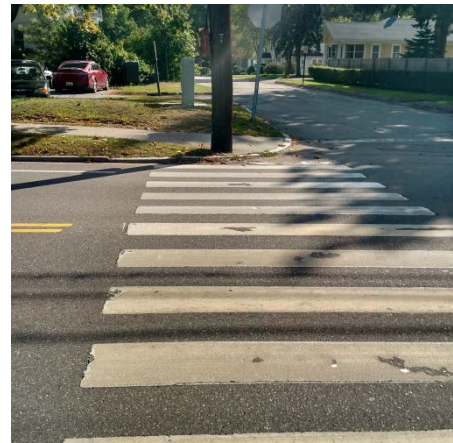
Figure 6. Crosswalk at Rossie Street Ending at Utility Pole
