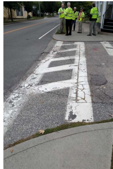
Figure 8. Crosswalk Across Isham Street
