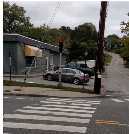
Figure 23. Lack of Pedestrian signal Heads
