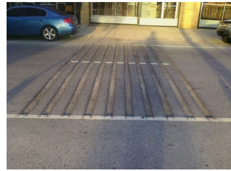
Figure 32. Passive Rumble Strips
