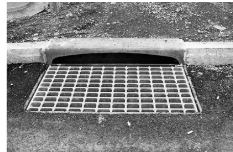
Figure 40. Bike Friendly Catch Basin Grate
