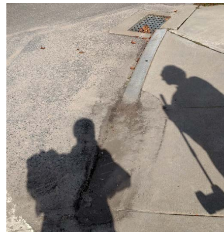
Figure 19. Sediment Build-up Due to Drainage Issue
