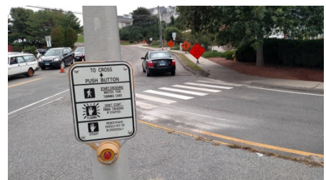
Figure 28. Unclear Which Crosswalk For Pedestrian Push Button
