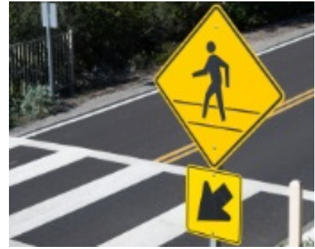
Figure 35. Advanced Warning Pedestrian Crossing Sign
