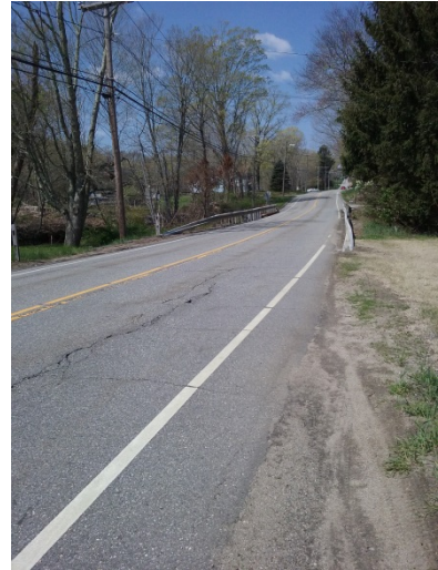
Figure 11. Merrick Brook Bridge
