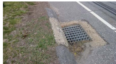
Figure 12. Bike Compliant Catch Basin
