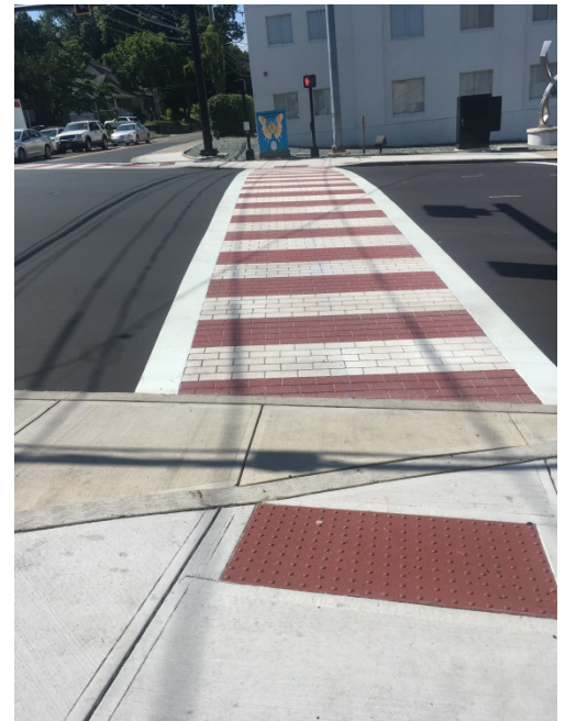
Figure 23: New stamped crosswalks
