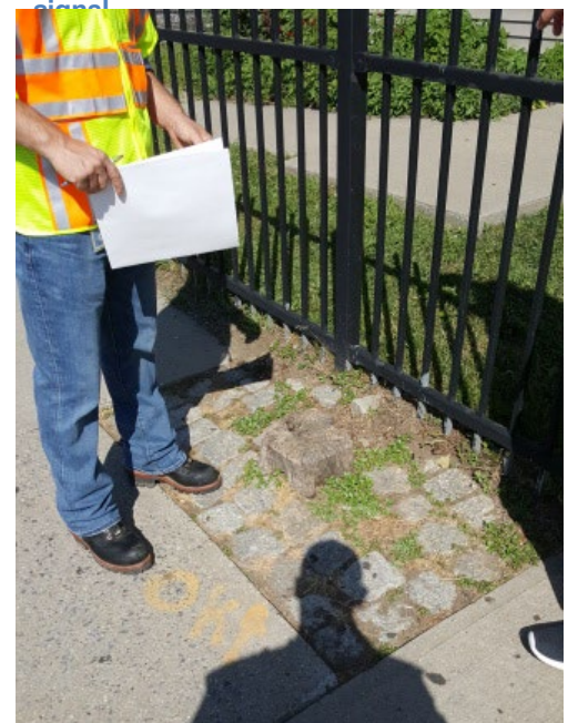
Figure 20: Tree trunk tripping hazard
