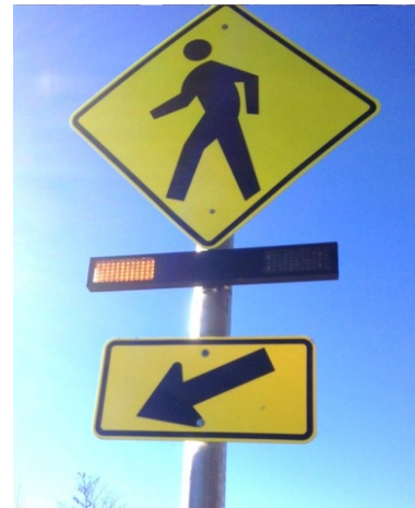
Figure 19. Rectangular Rapid Flashing Beacon
