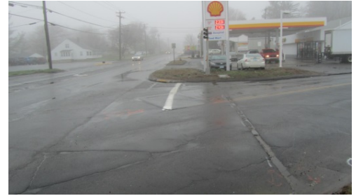
Figure 9: Route 69 northbound at Summit Road
