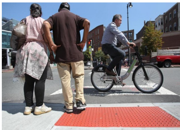
Figure 23. Example of Detectable warning Strips
