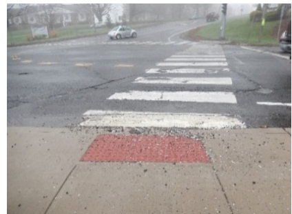
Figure 7: Crosswalks at Route 69/68 intersection
