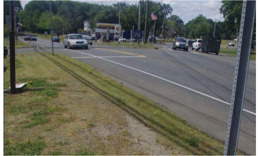
Exhibit 27: No sidewalks near the Ardsley Avenue intersection
