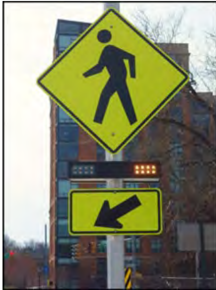
Exhibit 35: An example of RRFB (Source: CTDOT)
