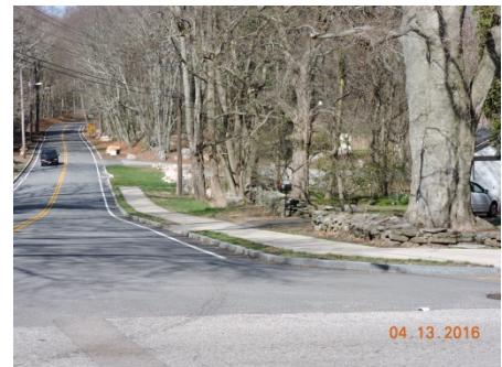
Figure 36. New Sidewalk Extension at Gallows Lane
