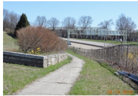
Figure 17. Lack of Pedestrian Wayfinding
