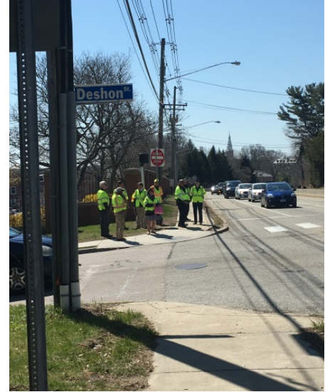
Figure 14. Lack of Sidewalk Across Deshon Street
