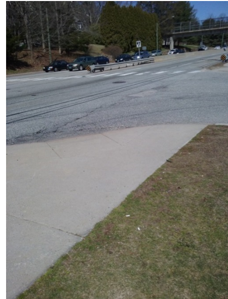
Figure 24. Lack of Traffic Calming
