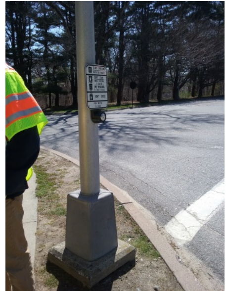
Figure 9. Push Button is not ADA Accessible
