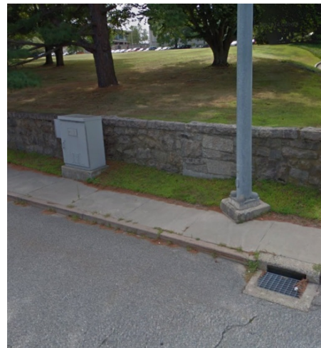
Figure 30. Span Pole in the Sidewalk
