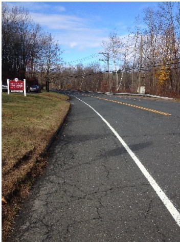
Figure 14: Route 44 looking north from crosswalk at Wickett Street (north)
