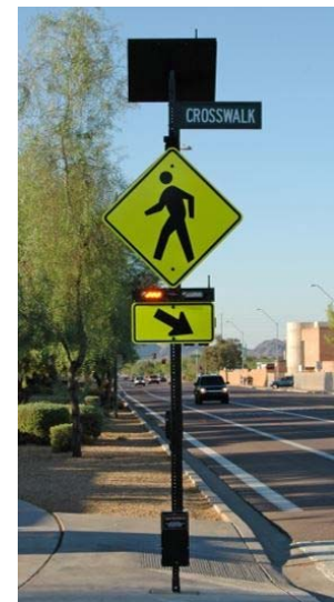
Figure 25: Rectangular rapid flashing beacon
