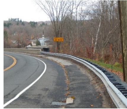
Figure 8: Sidewalk on east side of Route 44 looking north toward bridge
