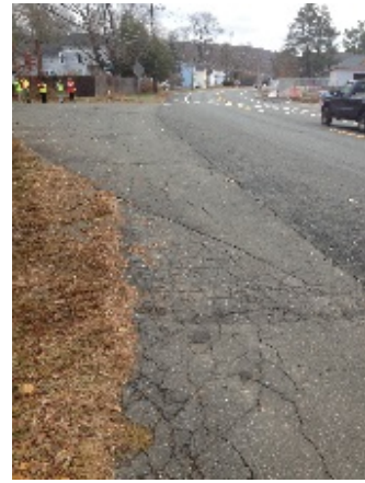
Figure 11: Looking south on Route 44 at Wickett Street (north)
