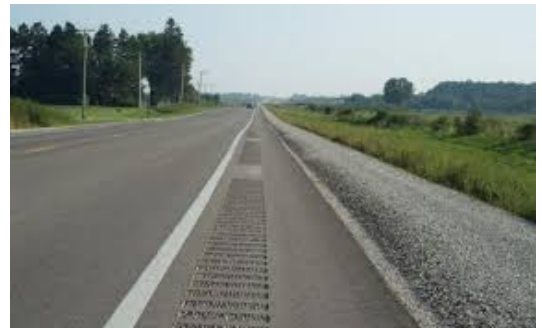
Figure 23: Shoulder rumble strips
