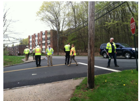
Figure 5. Sidewalk behind stop bar, no crosswalk, ramps or warning strips
