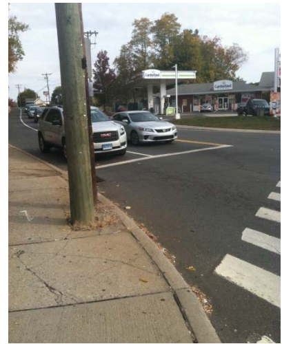
Figure 8. 10-foot shoulder on Meadow Street being used as a turn lane
