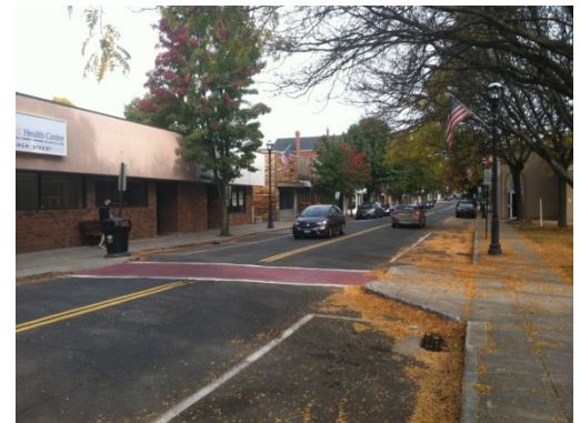
Figure 6. Mid-block crosswalk without pedestrian crossing signs
