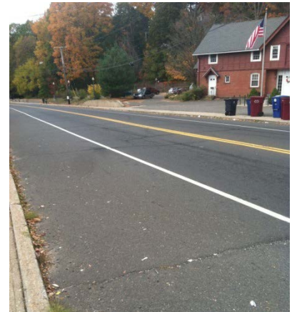
Figure 11. Wide shoulder/parking lane
