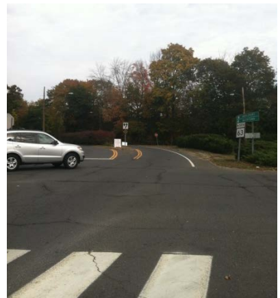
Figure 12. Missing crosswalks at intersection of Church Street and Meadow Street
