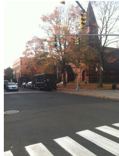
Figure 5. Church Street and Maple Avenue signal
