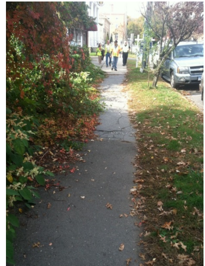
Figure 14. Vegetation growth onto sidewalk on Cedar Street
