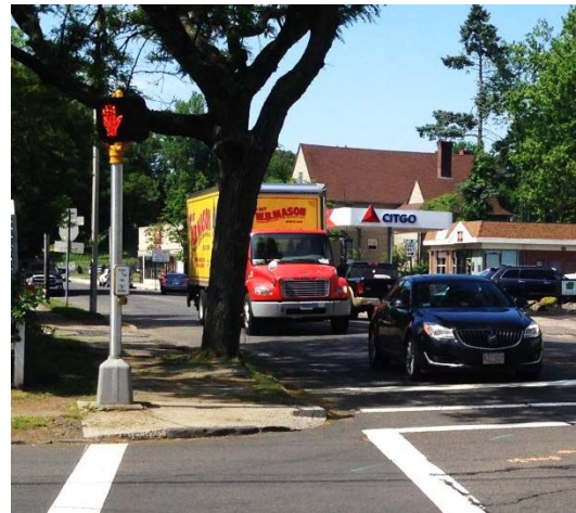
Figure 5. Tight Turns –No shoulder striping, No ADA Ramps.
