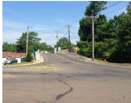
Figure 8. Steep grades on Camp St. Bridge
