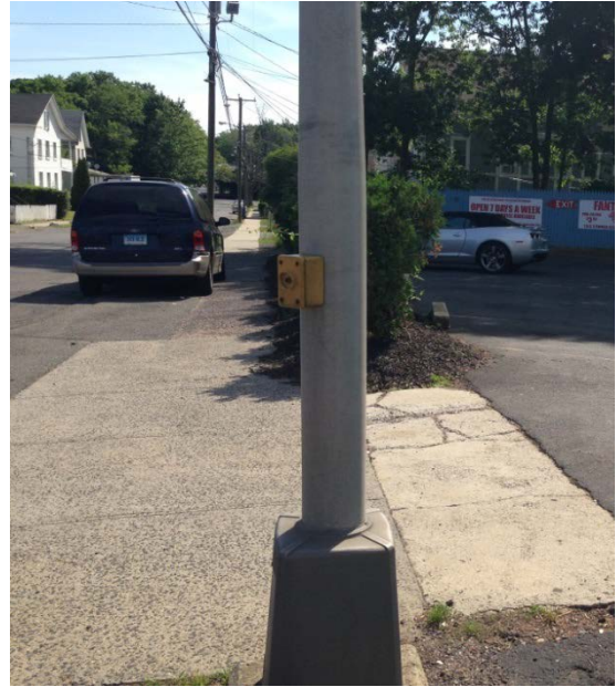
Figure 9. Insufficient clearance for Utility Poles
