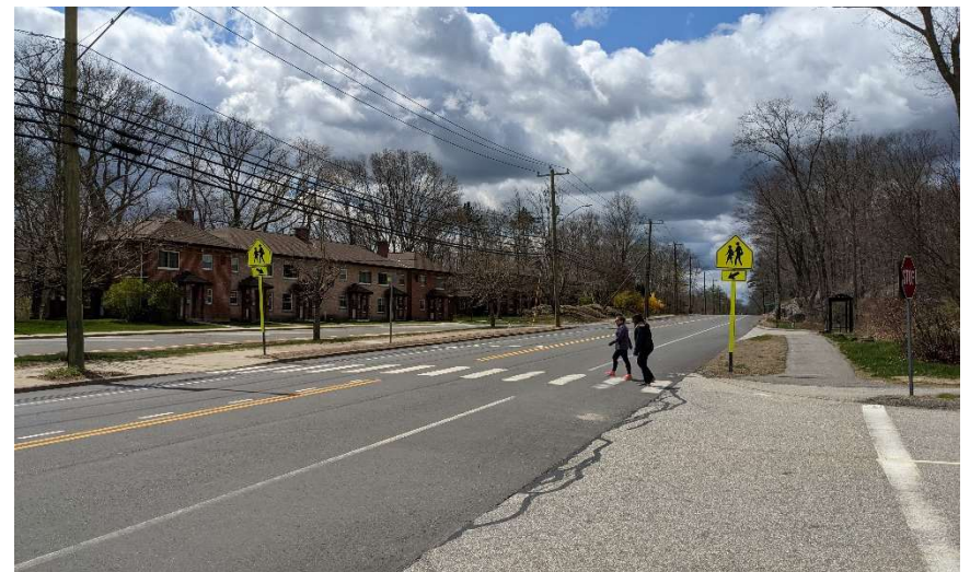
Exhibit 19: Crosswalk on Route 275 (South Eagleville Road) at Mansfield Community Center
