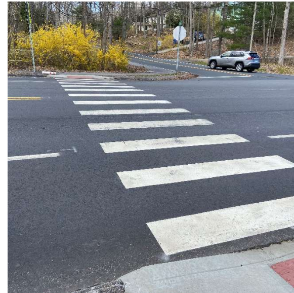
Exhibit 6: Crosswalk on Route 275 (South Eagleville Road)
