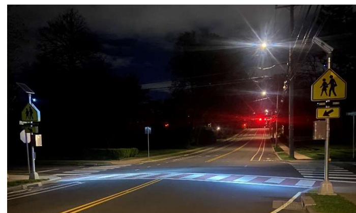
Exhibit 35: An example of a crosswalk high intensity light integrated with an RRFB at night in West Hartford, CT. Note – The yellow flashers are not activated in this photo to demonstrate the crosswalk light.
