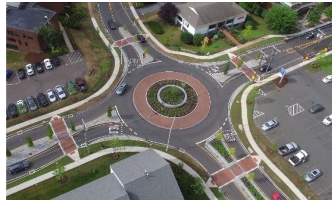
Exhibit 37: A modern roundabout in Glastonbury, CT serves a safer intersection control compared to a conventional signalized intersection 1 but also reduces vehicle travel speeds for motorists entering the town center. (Source: FHI Studio)
