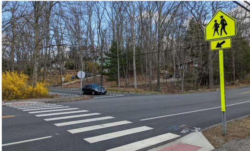
Exhibit 20: Crosswalk on Route 275 (South Eagleville Road) at Eastwood Road.
