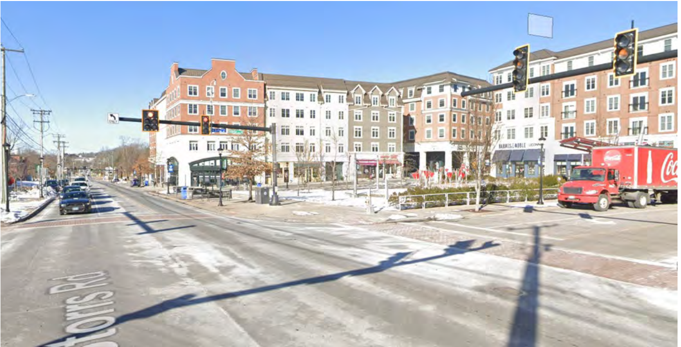
Storrs Center mixed use development. Image Credit: Google Street view
