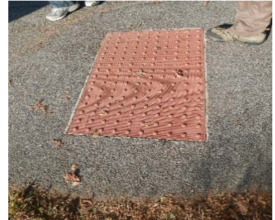
Figure 13: ADA compliant curb ramp
