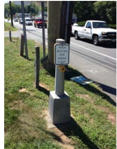
Figure 6. Pedestrian Button and Wide Shoulder on Route 154 Northbound Approaching Bridge Road
