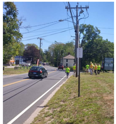
Figure 9. South Side of Bridge Road With Utility Poles
