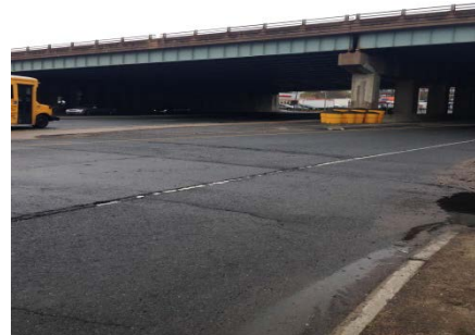
Figure 15. No Crosswalk on Ramp
