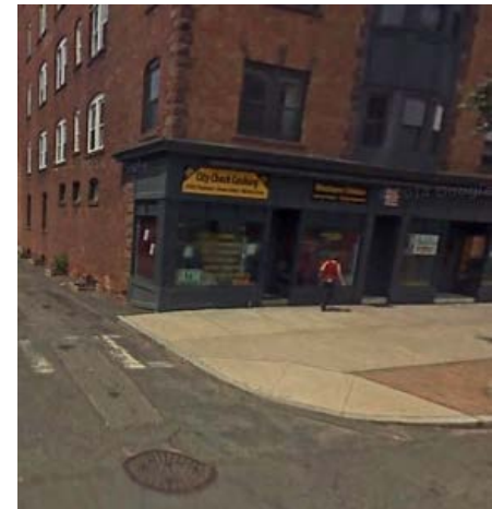
Figure 12. Misaligned Handicap Ramp at Roberts Court
