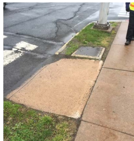
Figure 10. No Detectable Pedestrian Warning Strips at Rector Street
