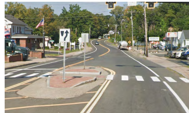
Exhibit 31: A crosswalk with pedestrian refuge island in Cheshire, CT allows pedestrians to cross in two-stages. (Source: Google Maps)
