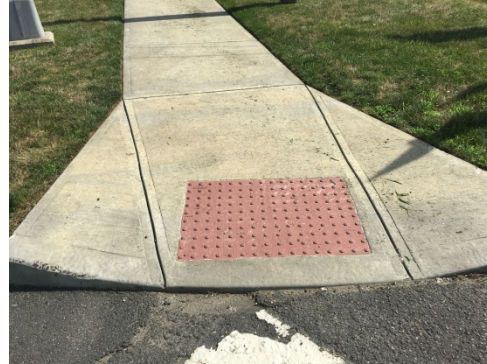
Figure 6. Detectable warning strip
