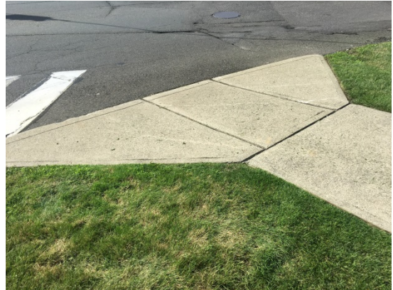
Figure 14. Ramp without detectable warning strip
