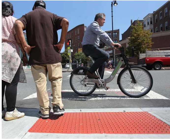
Figure 18. Ramp and detectable warning strip
