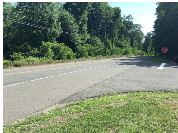
Figure 27. Construct sidewalk on Mill Plain Road
