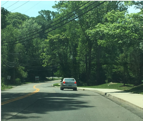
Figure 22. Paint shoulder lines on Saw Mill Road
