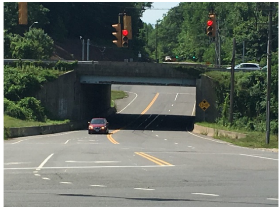
Figure 15. Bridge over Saw Mill Road
