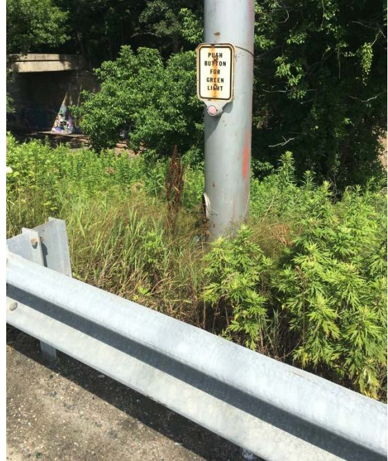
Figure 12. Inaccessible pushbutton
