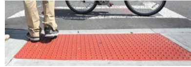
Figure 26. Example of Detectable Warning Strip
