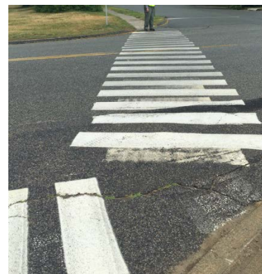
Figure 24. Square up Crosswalk
