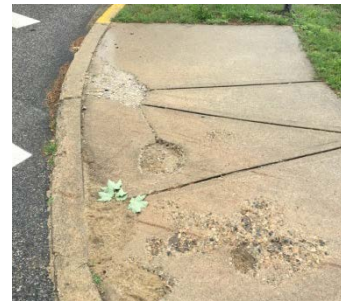
Figure 23. Repair Broken Ramp
