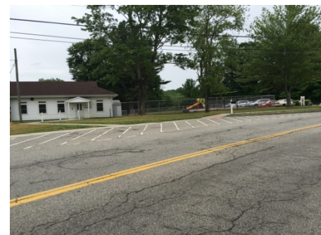
Figure 6. Pullout in Front of Daycare
