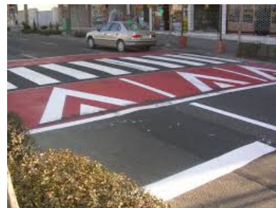
Figure 28. Speed Table
