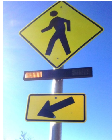
Figure 27. Example of Active Pedestrian Crossing Sign
