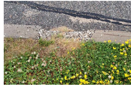
Figure 8. Broken Curbing
