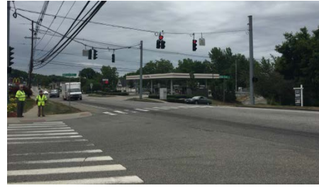
Figure 19. Route 85 and Halls Hill Road Intersection
