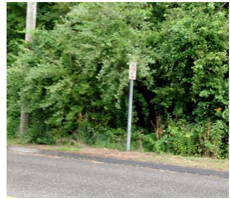
Figure 12. Sign Blocked by Vegetation
