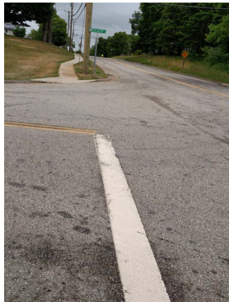
Figure 18. Lack of Crosswalk at Pleasant Street.
