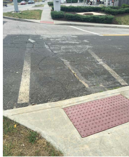
Figure 20. Crosswalk at Dr Foote Drive
