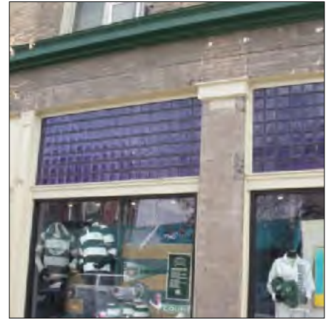
Glass block in transom of storefront
