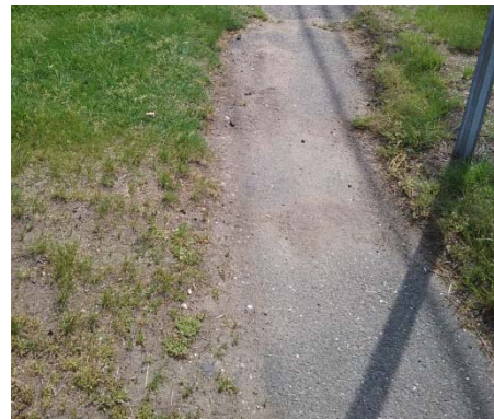
Figure 15. Narrow Asphalt Sidewalk
