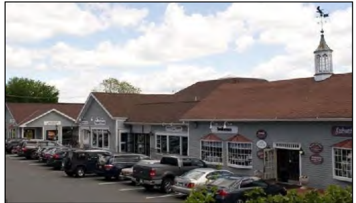
Small building shopping center (some attached) with parking
