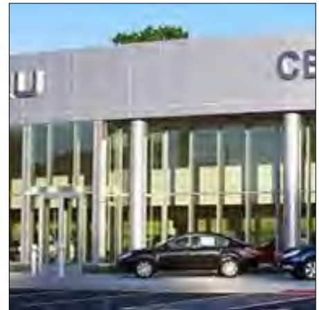
Glass curtainwall system
