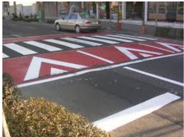
Figure 28. Example of Speed Table
