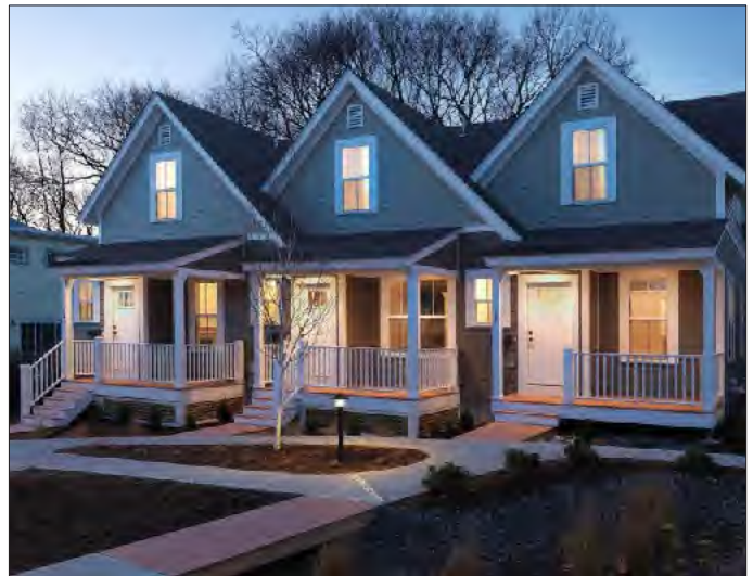
Attached single family “cottages”
