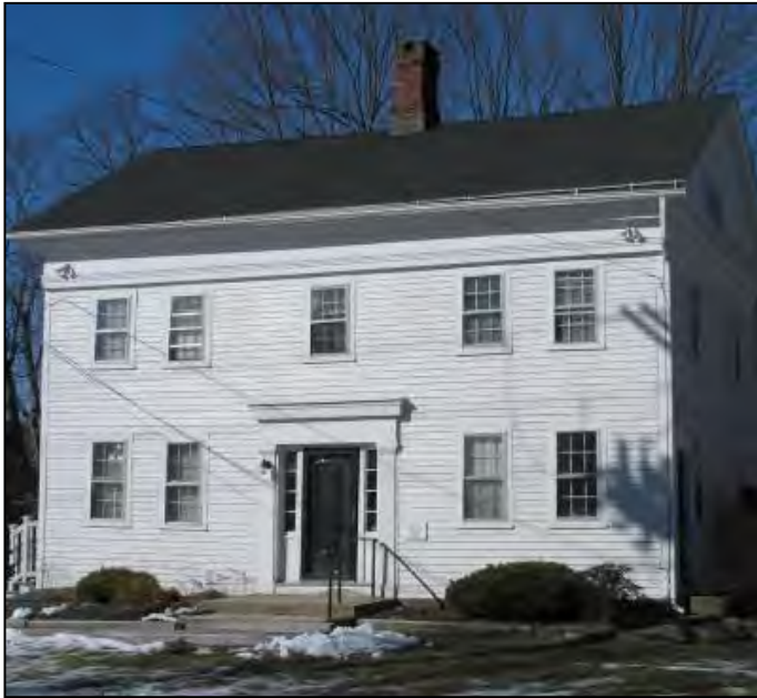
Simple, yet well detailed, wood siding
