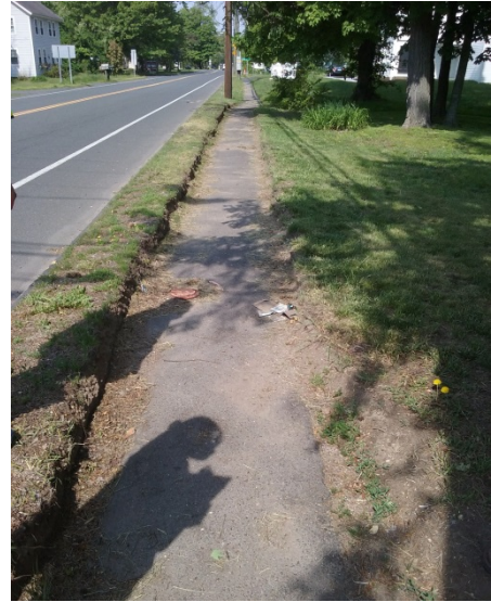
Figure 8. Recently Unearthed Sidewalk on Dowd Avenue
