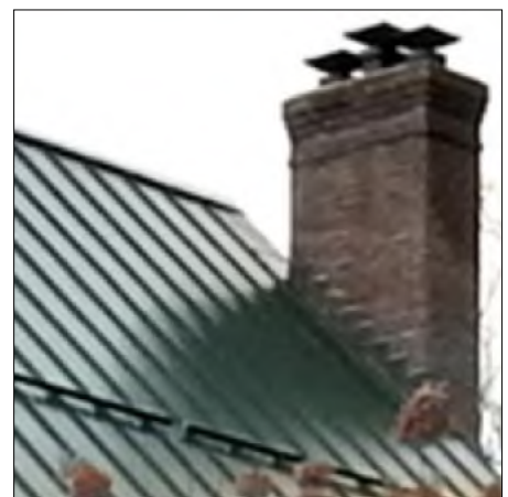
Standing seam metal with snow guards
