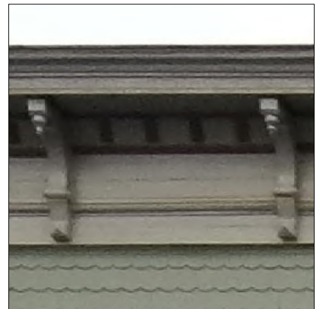
Projecting cornice at parapet
