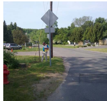
Figure 5. Poor Sight Distance From the Rail Trail Crossing
