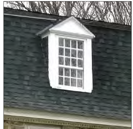
Dormer in asphalt shingle roof
