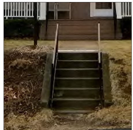
Planted embankment and grade change
