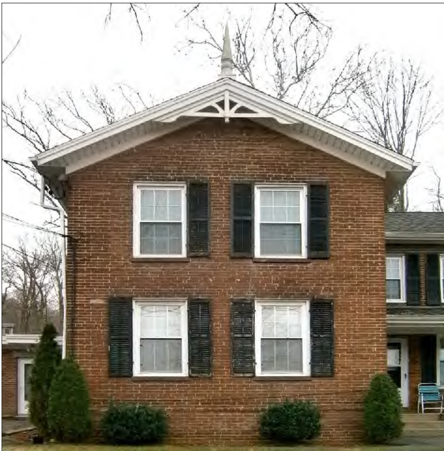
Eaves – projecting from the gable end of the building form – with decorative trim
