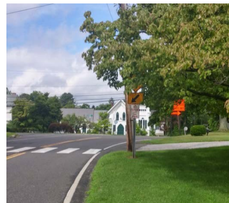
Figure 13. Pedestrian crossing sign blocked by branches on westbound Clapboard Road
