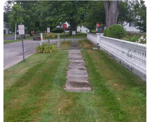
Figure 8. Existing granite sidewalk on Center Street
