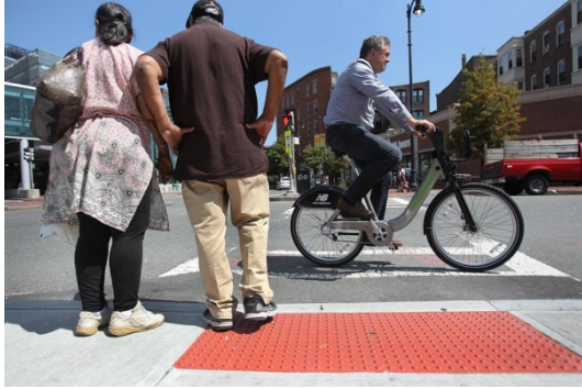
Figure 23. Pedestrian detectable warning strip
