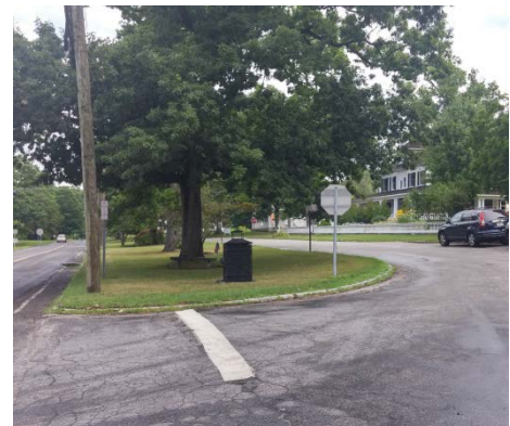
Figure 7. Stop sign on Center Street set back from stop bar
