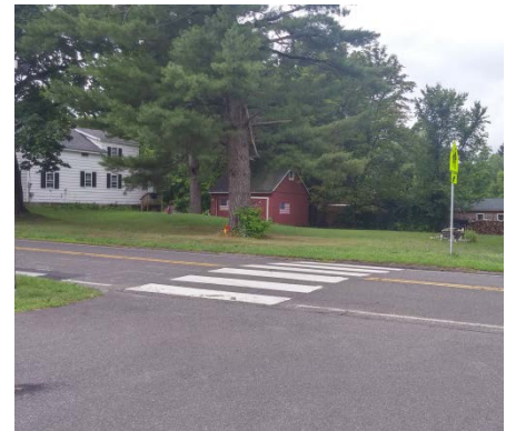
Figure 18. Burnham School (south) driveway crosswalk
