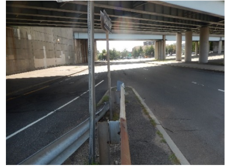
Figure 13. Route 8 Off-ramp and Main Street Merge
