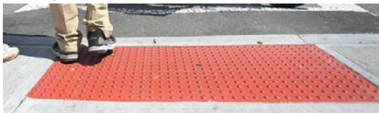
Figure 28. Example of Tactile Warning Strips
