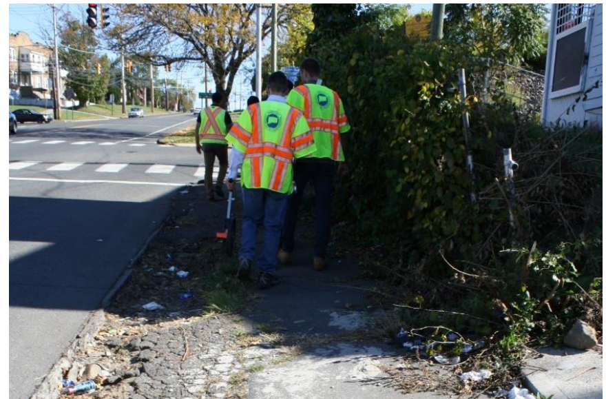
Exhibit 26: Sidewalks in poor condition in the vicinity of Central Avenue
