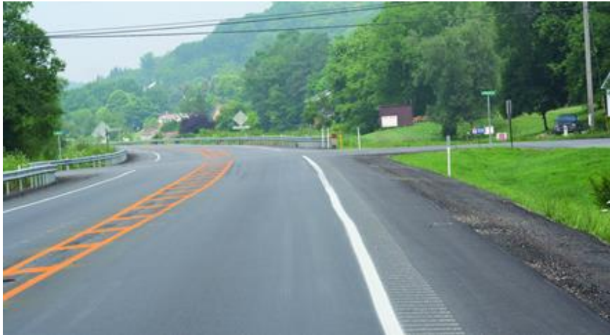
Exhibit 34: Example of travel lane narrowing with the installation of a painted median (Source: Federal Highway Administration)
