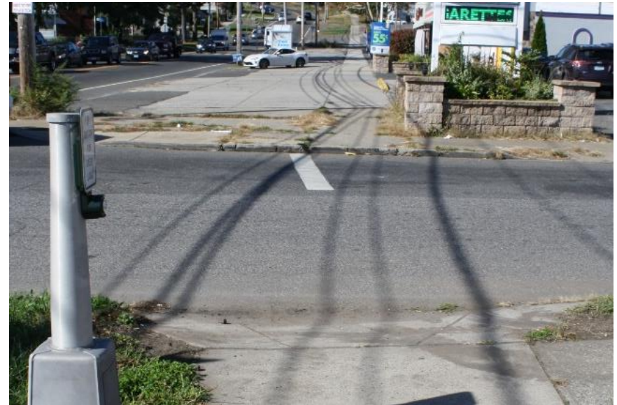
Exhibit 19: Missing crosswalk and confusing crossing environment at the intersection of Route 1 and Success Avenue
