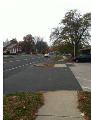
Figure 13. Several driveways close together
