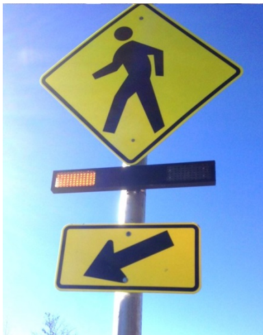
Figure 16. Rectangular Rapid Flashing Beacon (RRFB)
