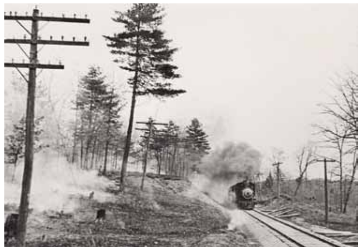
Sparks from trains were once a significant cause of fires in Connecticut, as seen in this photo (date unknown).
